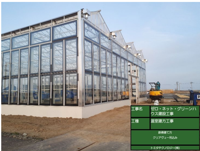
Partially glazed greenhouse at Aqua Ignis Sendai showing installed ClearVue PV IGU panels of custom dimension - 1.908m high x 0.95m wide.
