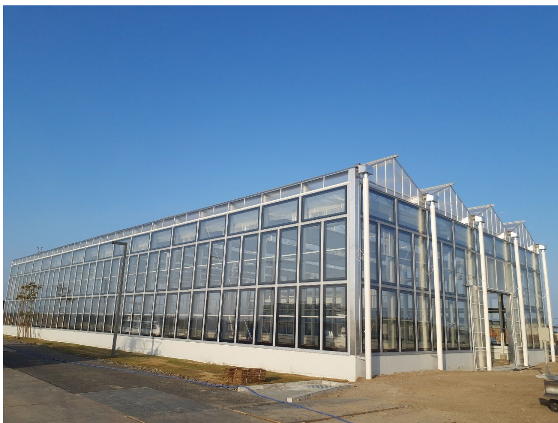
Partially glazed greenhouse at Aqua Ignis Sendai showing installed ClearVue PV IGU panels of custom dimension - 1.908m high x 0.95m wide.
