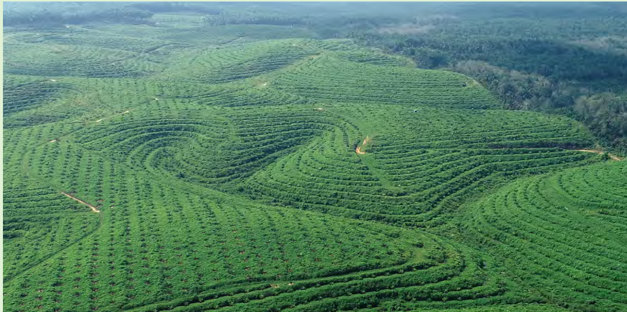
Planning and monitoring of terracing work in the replanting at Sei Rumbiya Estate via drone Perencanaan dan pemantauan pekerjaan terasering menggunakan drone di Sei Rumbiya Estate replanting
