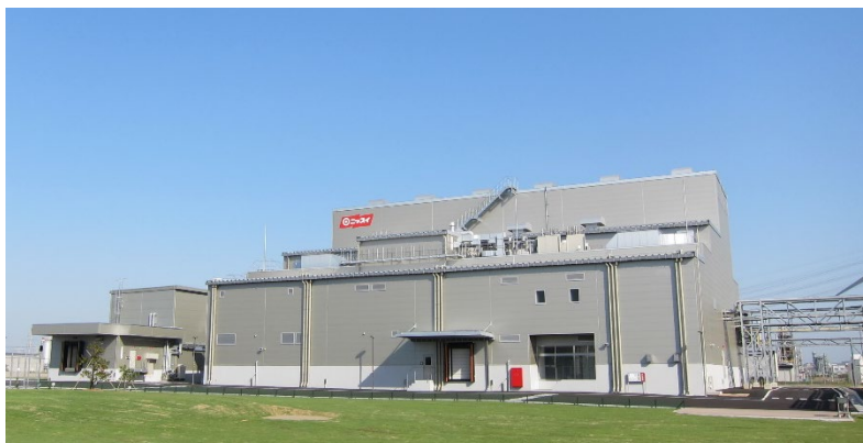
Fine Chemicals General Factory Kashima Pharmaceutical Factory Completed on May 11, 2017
