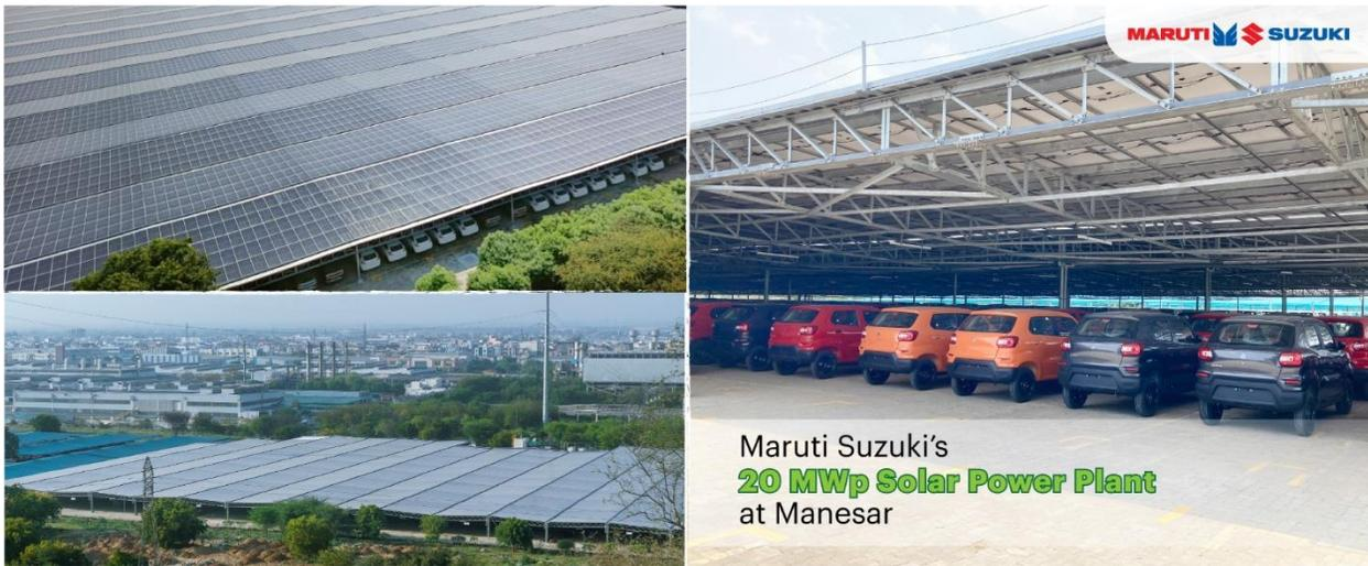
\*A solar carport is an overhead shade designed as parking area shelter with solar panels mounted on them.
