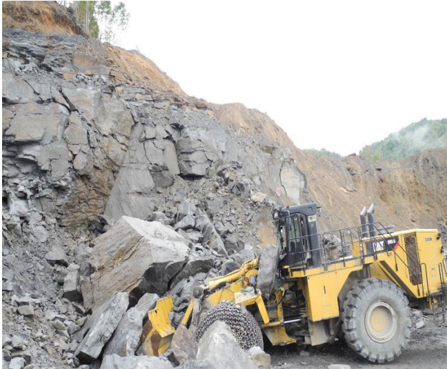
A FEL operator was seriously injured when a section of highwall fell onto the CAT 992K FEL while operating next to a highwall.
