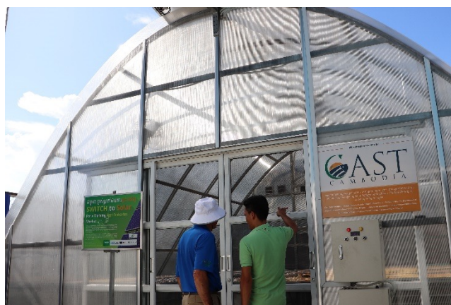
A solar dryer dome at a project beneficiary site, Samnang Sothea Fish Enterprise, used to reduce production costs and increase food safety. Photo credit: CAST Staff.
