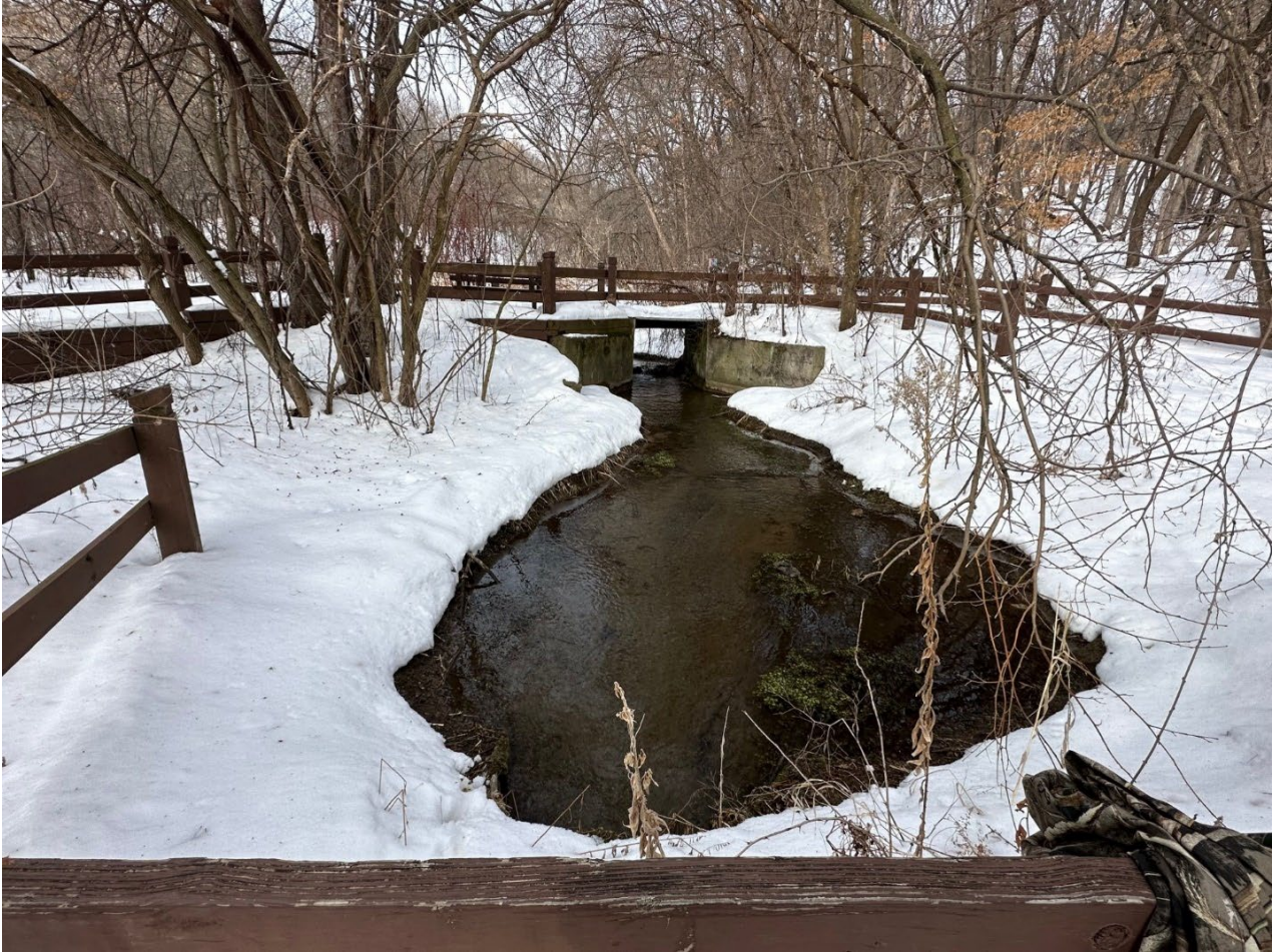
Figure 3: Water control structure
