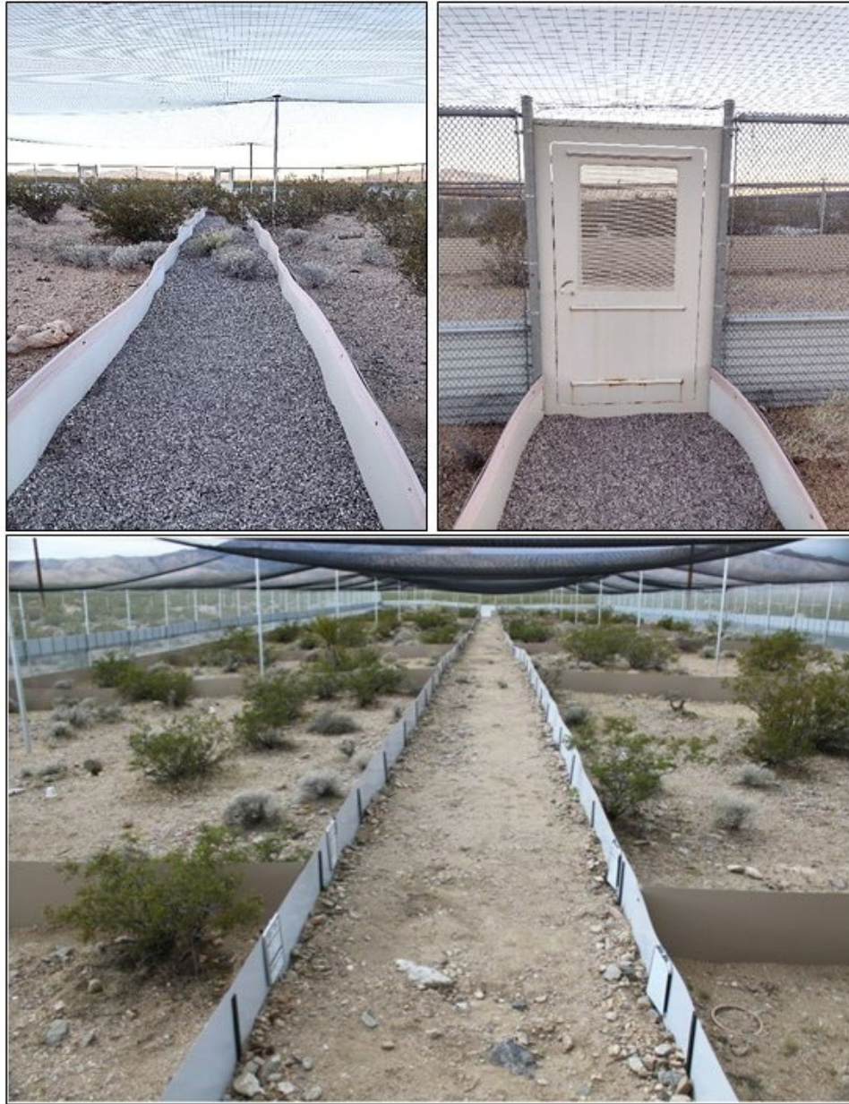
Figure 2. Examples of walkways between Mojave desert tortoise enclosures and secure points of entry or egress. Walkways are at least 1 m (3 ft.) wide and allow access to each enclosure without entering. Walkways lead to secure access points that are predator-proof. Photos courtesy of Ecocentric and the Ivanpah Desert Tortoise Research Facility.
