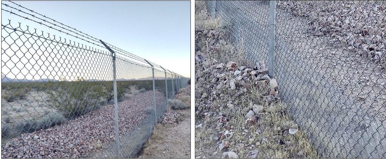
Figure 1. Example perimeter and security fencing for Mojave desert tortoise captive enclosures. Perimeter fencing is buried in the ground at least 30 cm (1 ft.) with the bottom flared outward to reduce wildlife digging. (Left) Chain-link fencing roughly 2.4 m (8 ft.) high with razor wire or strands of barbed wire at the top for additional security. (Right) Tortoise exclusion fencing attached to the bottom of chain-link fencing. Photos courtesy of the Ivanpah Desert Tortoise Research Facility.
