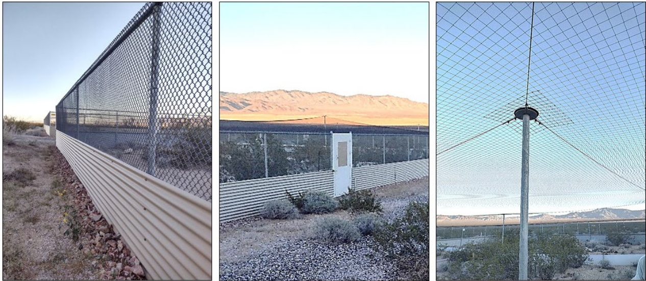
Figure 6. Examples of predator-proof enclosures for Mojave desert tortoises. (Left) Rodent-proof flashing attached to the bottom of a chain-link fence walk-in enclosure. (Middle) Secure access door to a walk-in enclosure with rodent-proof flashing bordering the door and predator-proof netting above the structure. (Right) Predator-proof netting over a walk-in enclosure. Photos courtesy of the Ivanpah Desert Tortoise Research Facility.
