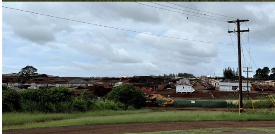
Hōkūau Residential Development under construction
