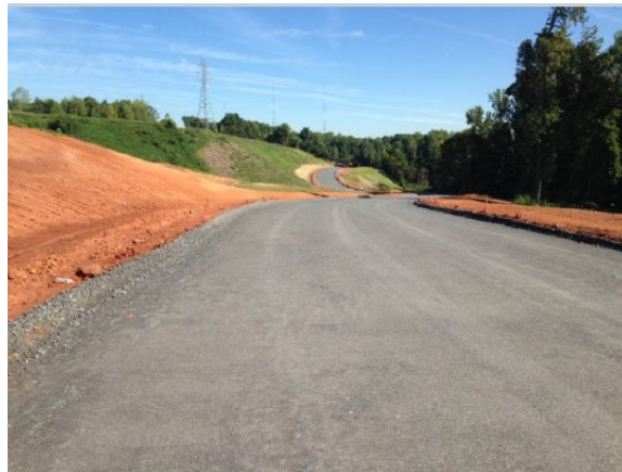
Figure 107. Photo. Unbound granular base construction; Quarry Access Road, North Carolina (Vaughan 2017).
