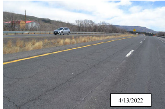
Figure 66. Photo. Longitudinal construction joint cracking in the northbound (left) and southbound (right) lanes; I-25, Colfax County, New Mexico.
