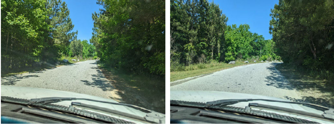
Figure 139. Photo. South African inverted pavement in the inbound lane in May 2022; Morgan County Quarry Access Road, Georgia.
