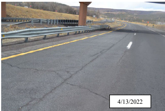
Figure 67. Photo. Transverse thermal cracks in the passing lane of the northbound section; I-25, Colfax County, New Mexico.
