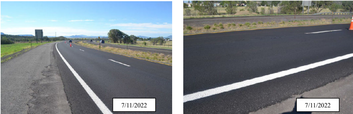
Figure 69. Photo. Northbound lanes after the overlay; I-25, Colfax County, New Mexico.
