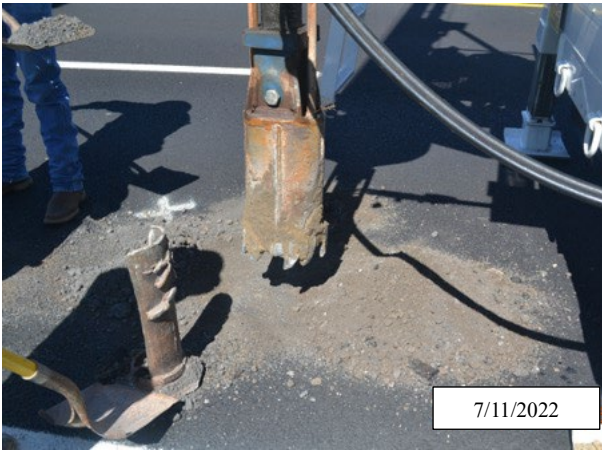
Figure 71. Photo. Boring operation and sampling of the cement-treated and granular base layers; I-25, Colfax County, New Mexico.
