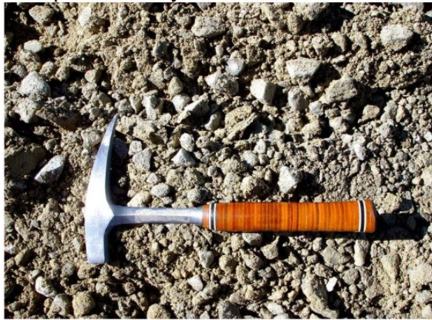
A. Loose G1 unbound aggregate base course material.
