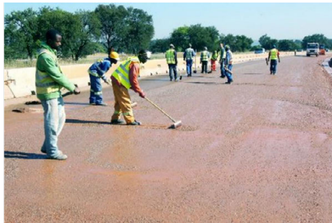
B. Brooming and spreading initial slush/fines to deficient areas.
