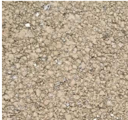
Figure 157. Photo. Dense-graded unbound dolomite aggregate layer construction in Cell 3 (Qamhia 2019).
