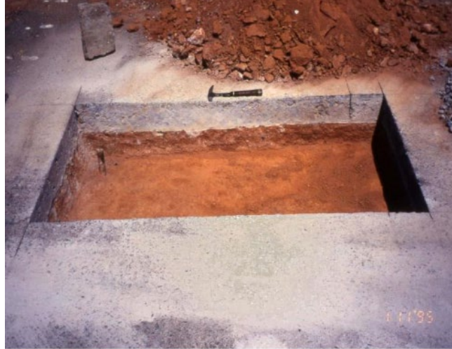
B. Constructed G1 base layer cut like concrete.
