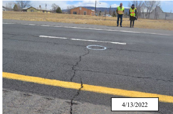
Figure 67. Photo. Transverse thermal cracks in the passing lane of the northbound section; I-25, Colfax County, New Mexico.
