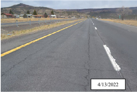
Figure 66. Photo. Longitudinal construction joint cracking in the northbound (left) and southbound (right) lanes; I-25, Colfax County, New Mexico.
