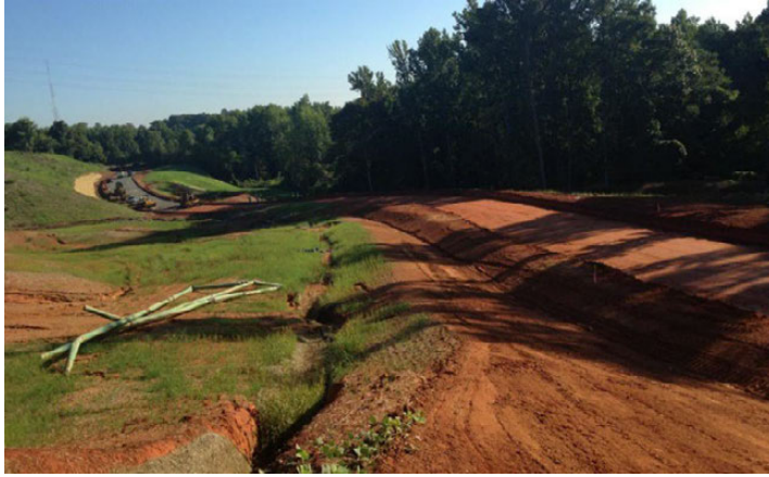
Figure 105. Photo. Subgrade; Quarry Access Road, North Carolina (left photo from Vaughan 2017).
