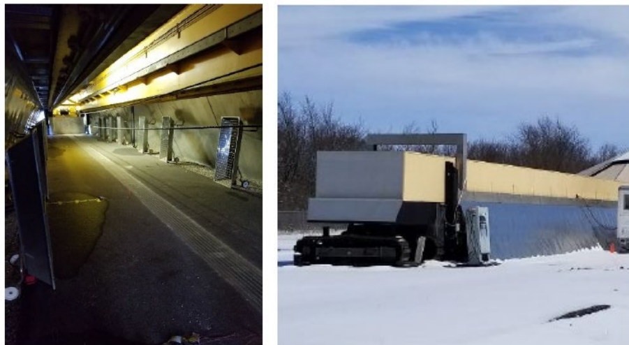
Figure 160. Photo. Insulation panels and heaters; ICT (Qamhia 2019).
