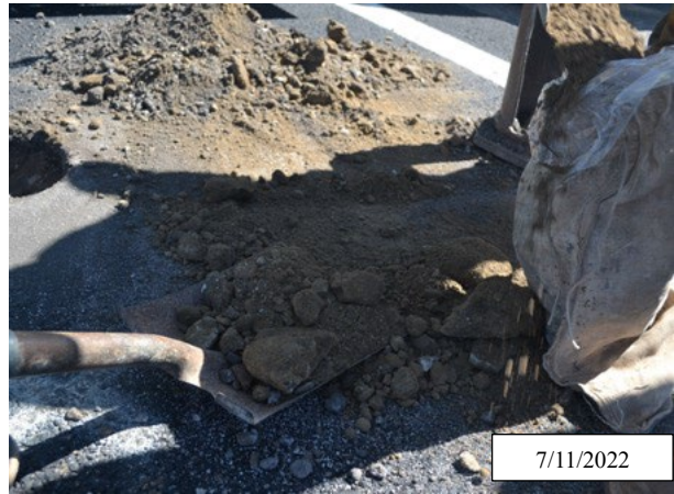
Figure 71. Photo. Boring operation and sampling of the cement-treated and granular base layers; I-25, Colfax County, New Mexico.
