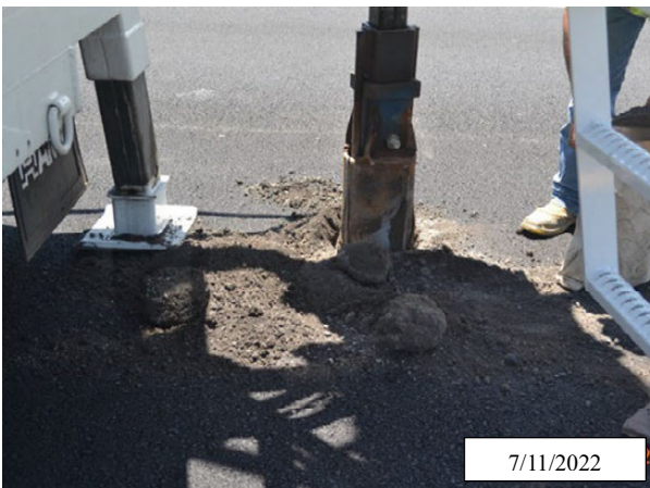
Figure 78. Photo. Cement-treated base layer materials extracted from both directions; I-25, Colfax County, New Mexico.
