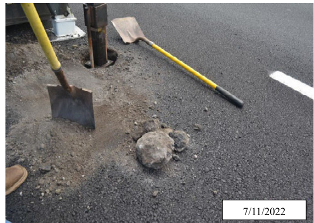
Figure 78. Photo. Cement-treated base layer materials extracted from both directions; I-25, Colfax County, New Mexico.
