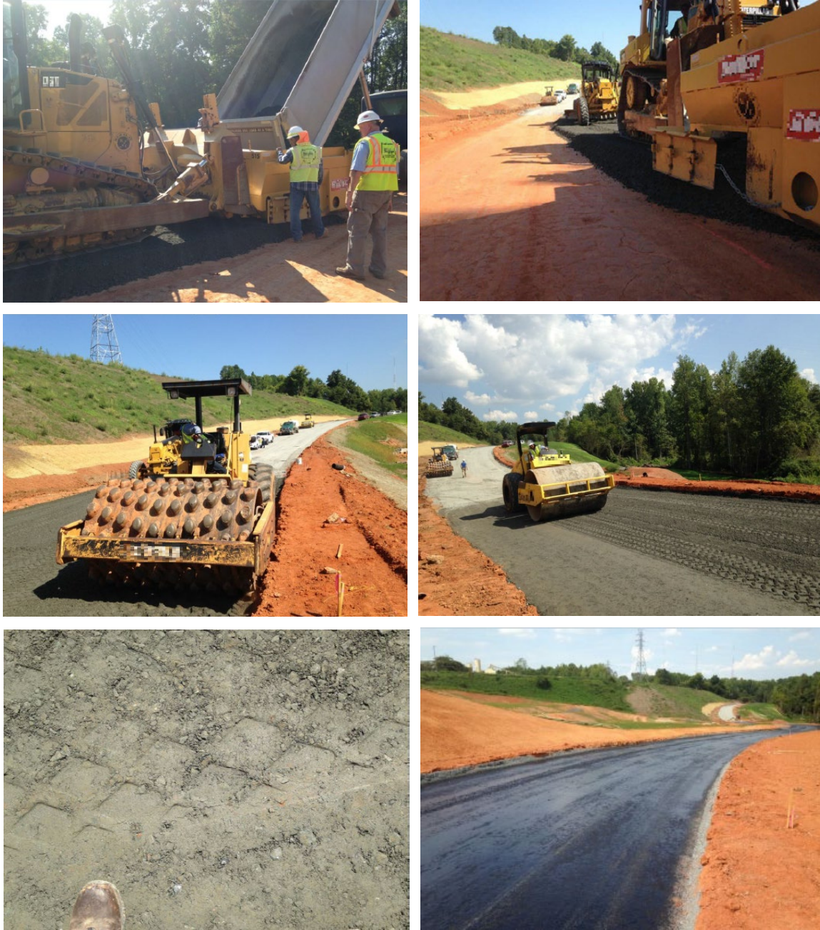
Figure 106. Photo. Cement-treated base construction; Quarry Access Road, North Carolina (Vaughan 2017).
