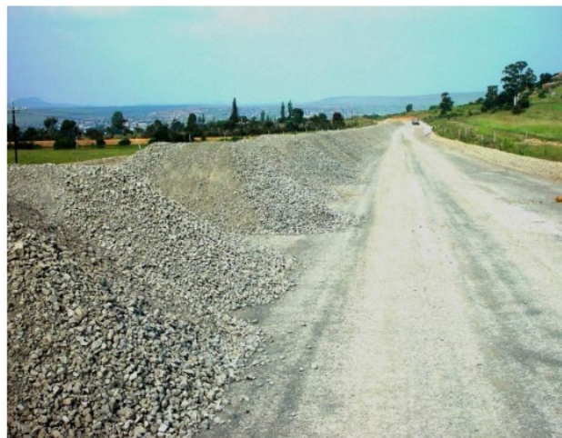
B. G1 material stockpiled along the road.
