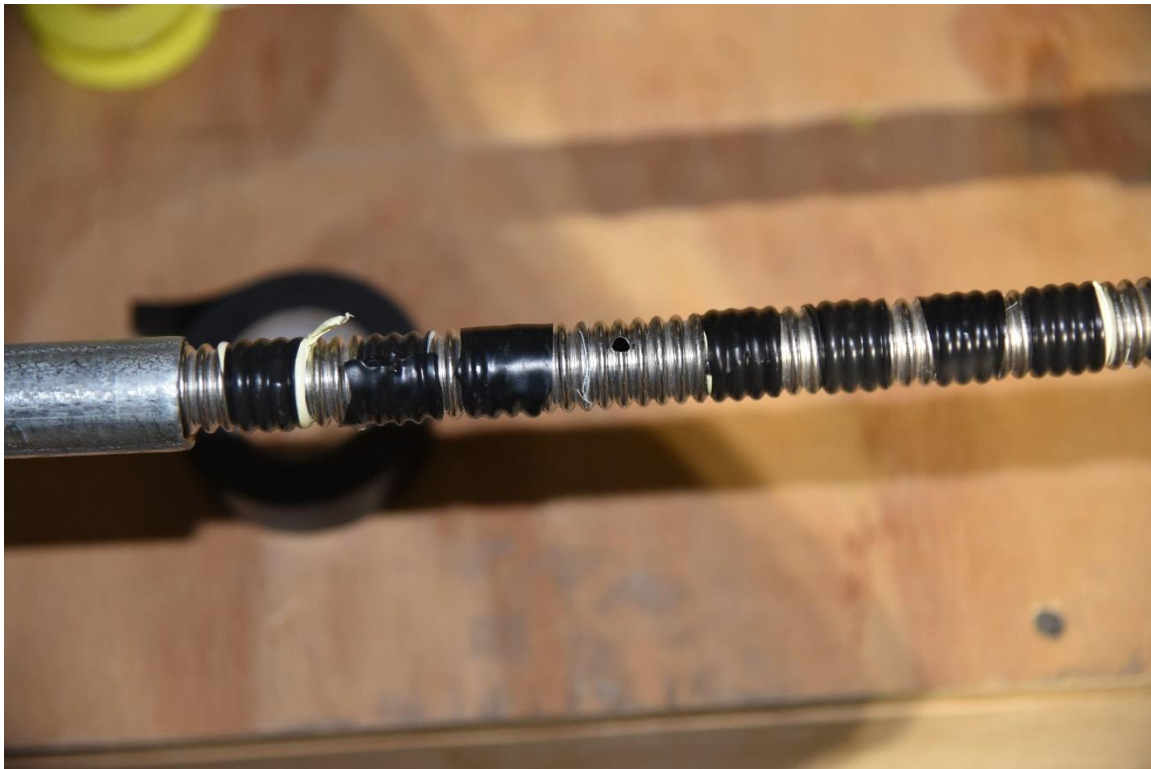
Figure 4. CSST test section (348035_1191808.jpg)
