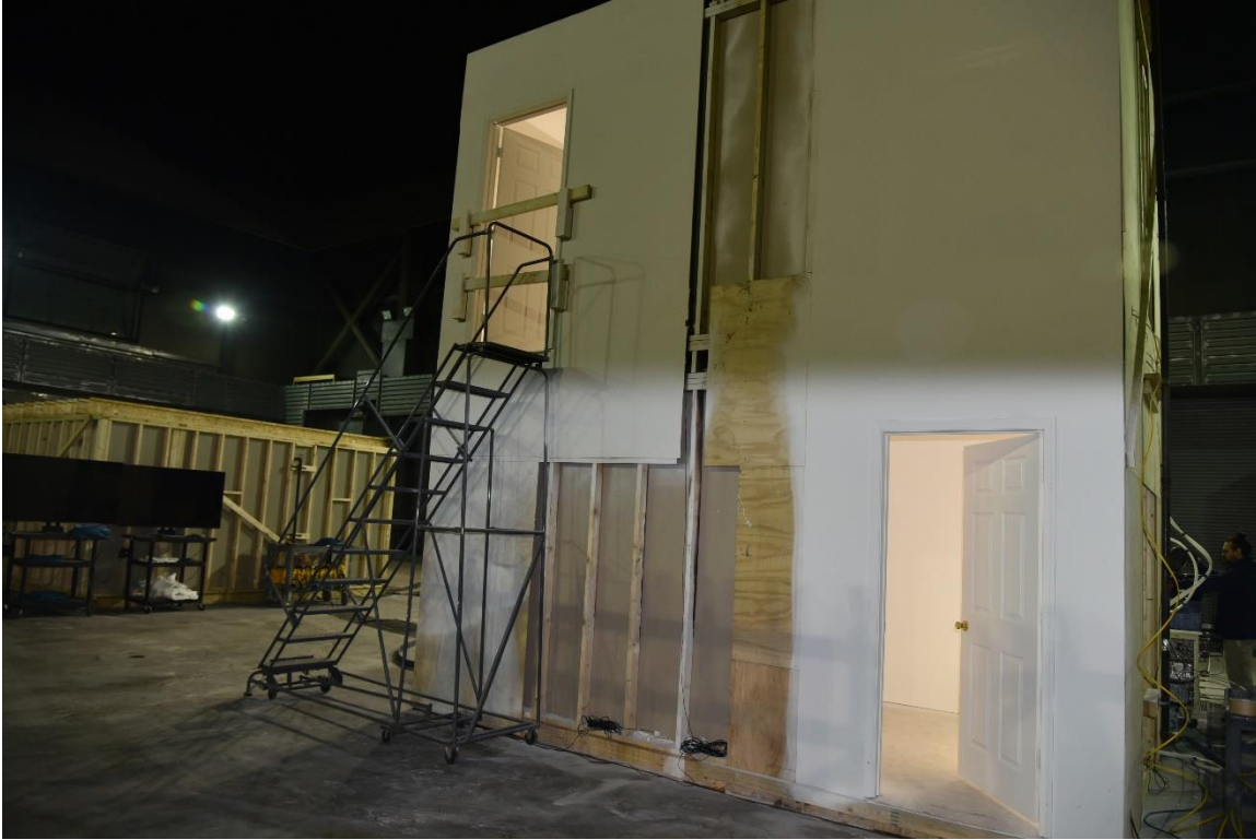
Figure 2. Exterior view of the east side of the structure (360079_1304634.jpg)
