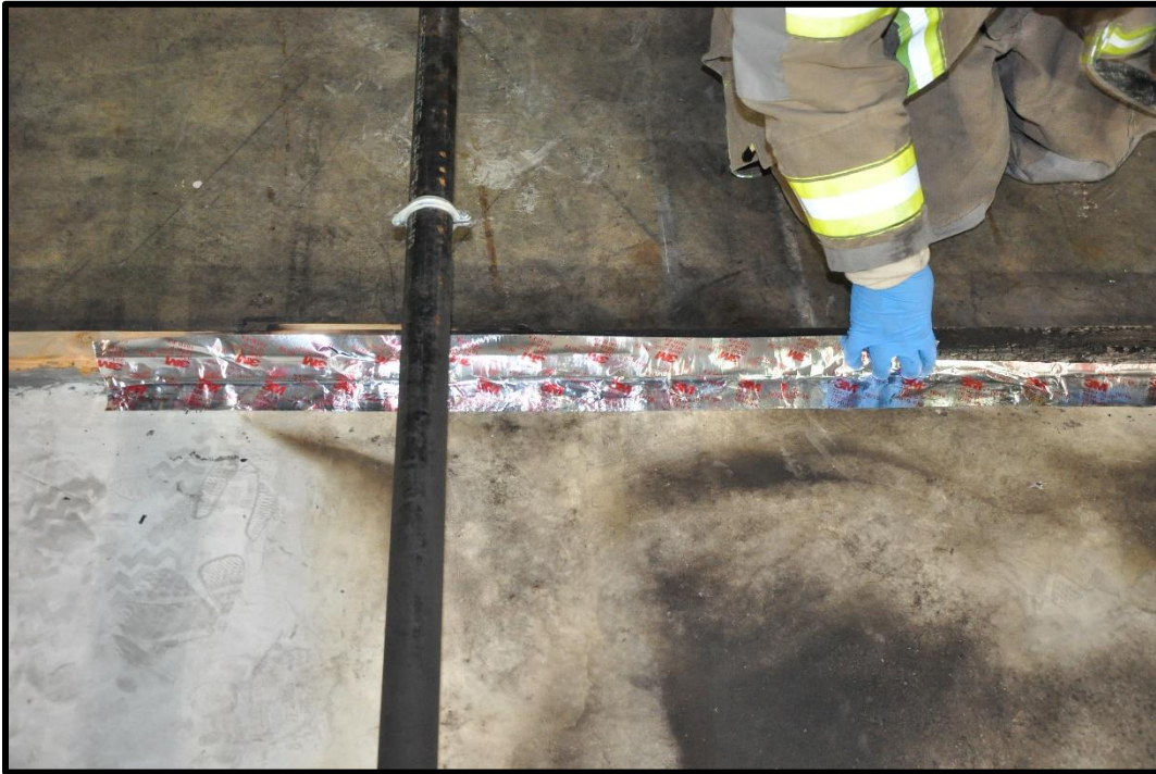
Figure 16. Foil tape being placed over gap between the pad and framing for Test # 4 (326955_1121074.jpg).
