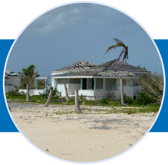
Photo: Storm damaged beach on the island of Barbuda.
