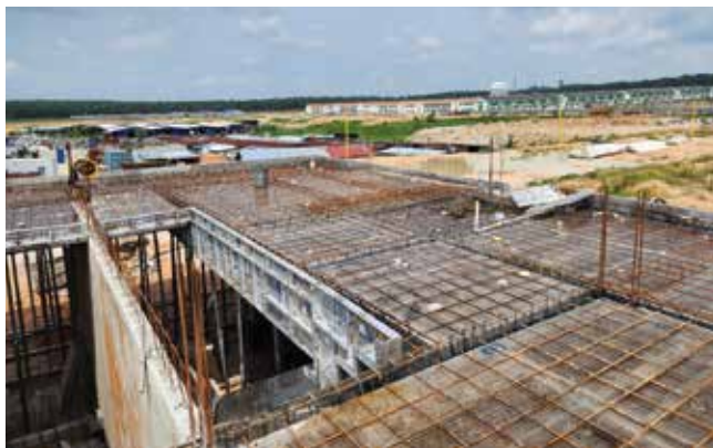
A sample development utilising aluminium formworks
