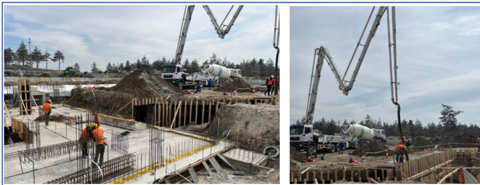
Figure 3. View from construction works of the WHR facility
