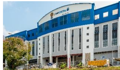
11 Changi South Street 3
