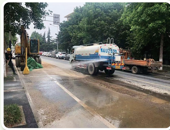
A Sprinkler Flushes the Road to Control Dust
