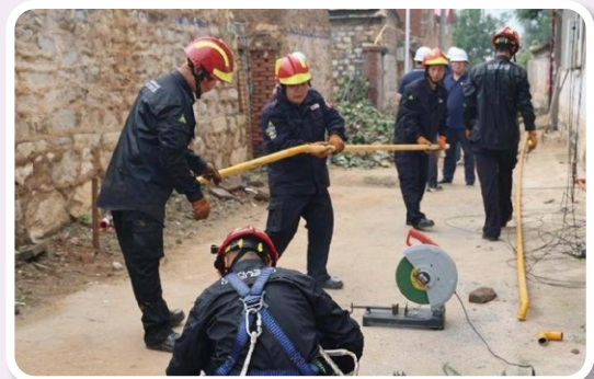
Gas Workers Repairing Coal-to-Gas Pipelines
