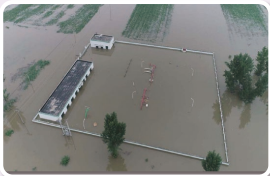
Drone Inspection at Beiliuzhuo Gas Station in Baoding City
