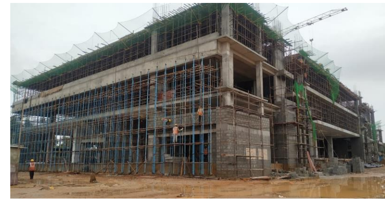
Above: Construction as at August 2022
