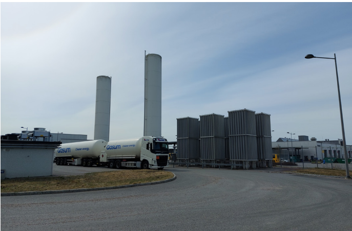
Uppsala Vatten also operates a plant that converts liquefied natural gas (LNG) and liquefied biogas (LBG) back into a gaseous aggregate state. Photo: OST
