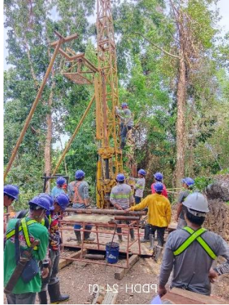
Drill rig setup
