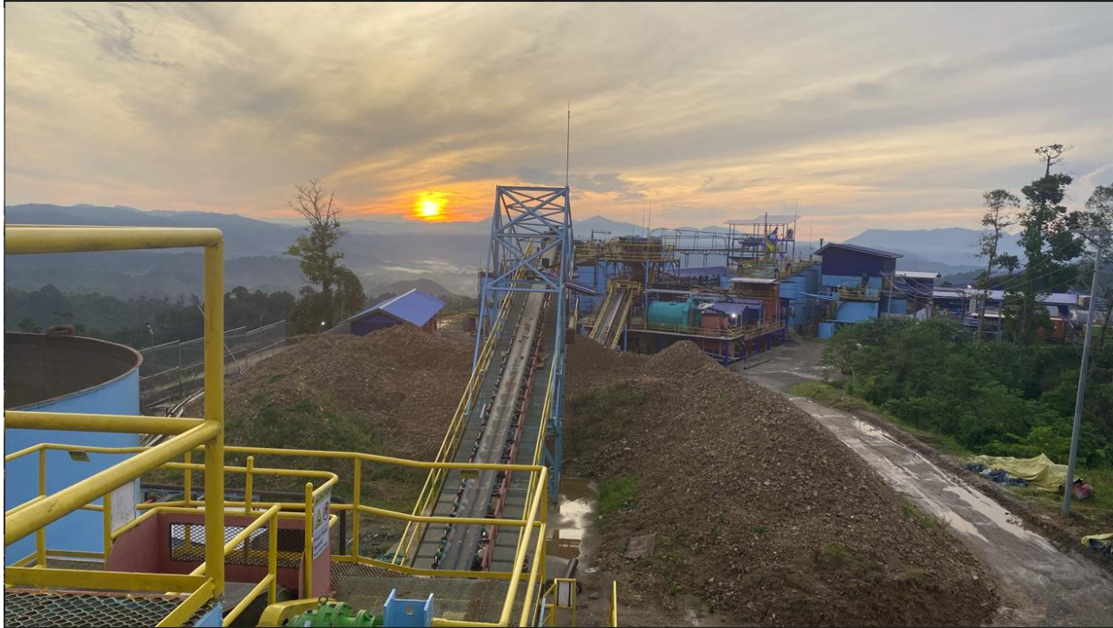
Balabag Gold & Silver Project process plant (June 23, 2024)
