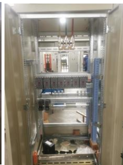
MCC CABINET CENTRE & ONE WITH DOOR OPEN
