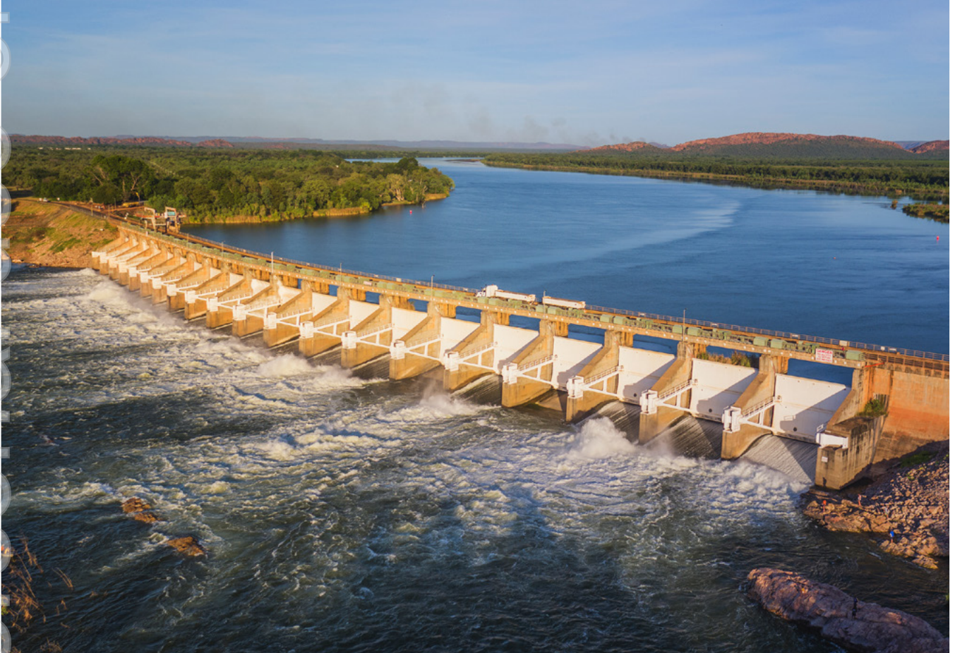
Diversion Dam, Kununurra. Photo Credit: Ben Broady
