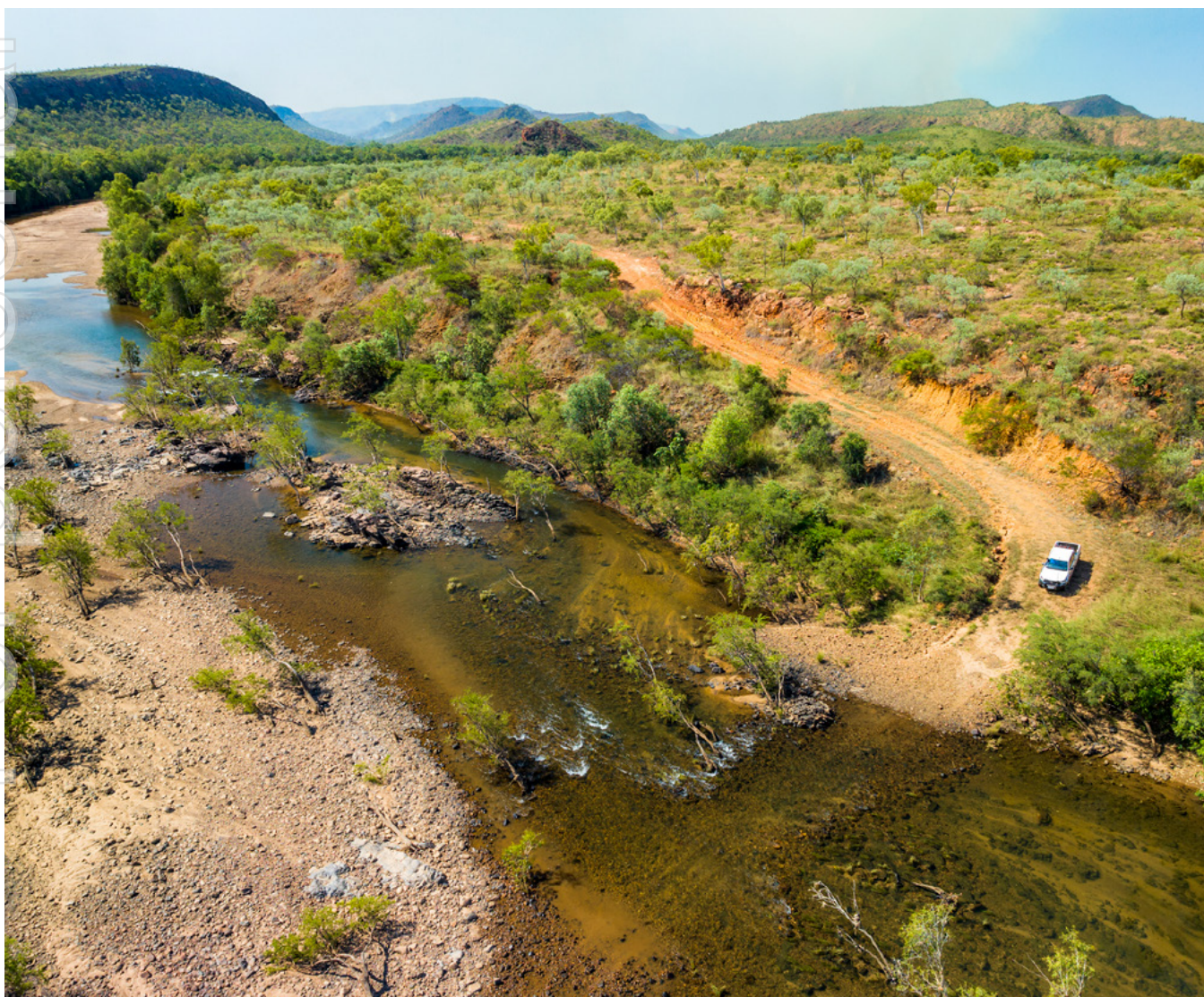
Figure 46: Photo of the existing historical tracks at the Dunham River Crossing, demonstrating nature of the existing terrain, and access track interaction with primary, secondary and tertiary watercourses. Photo Credit: Ben Broady
