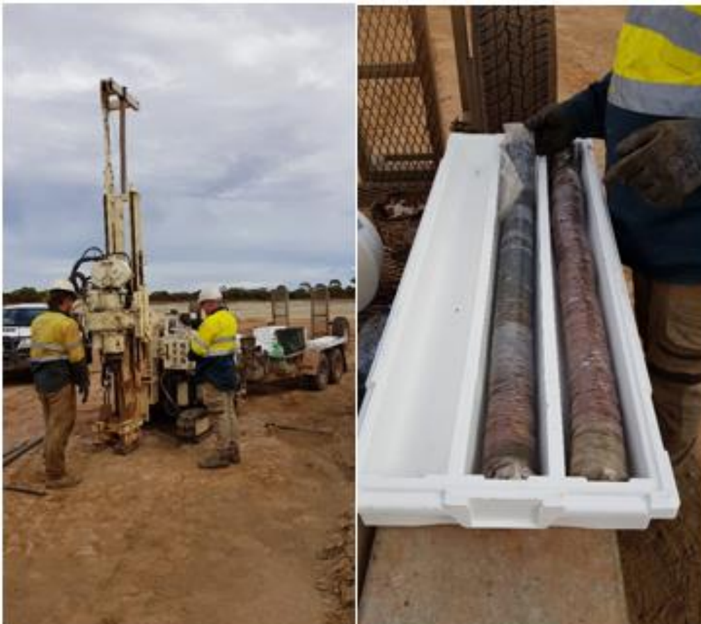
Figure 2: Sonic rig drilling on SST dam (left) and example of sonic 'core' (right)
