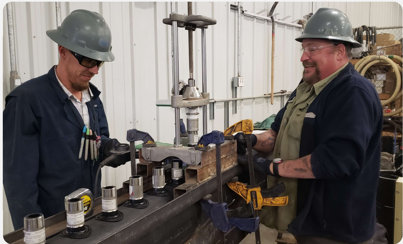
Fabricating Piping Segments in the Lance Construction Shop
