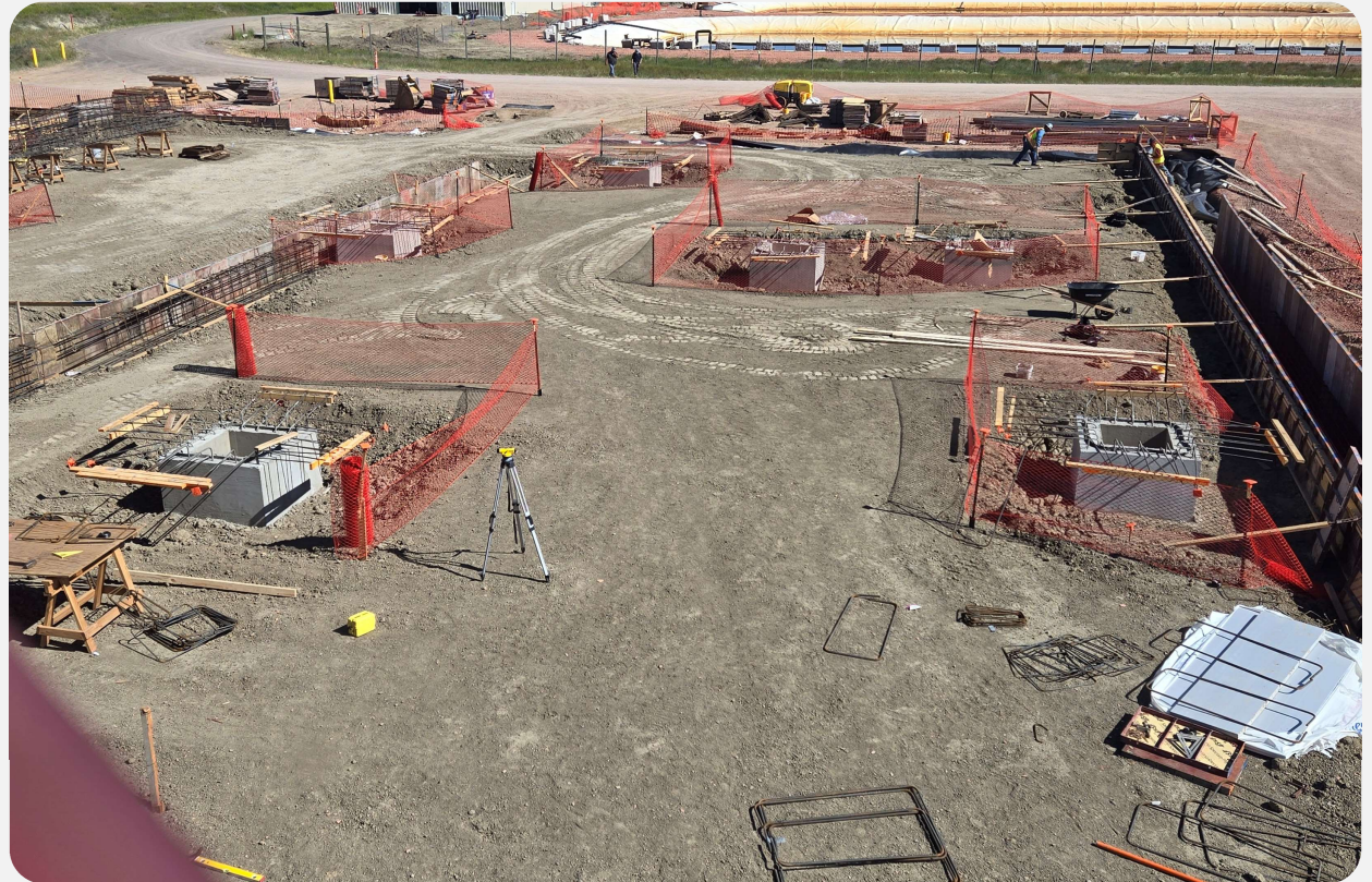
Lance Central Processing Plant Site: Early July 2024 - Subgrade preparation
