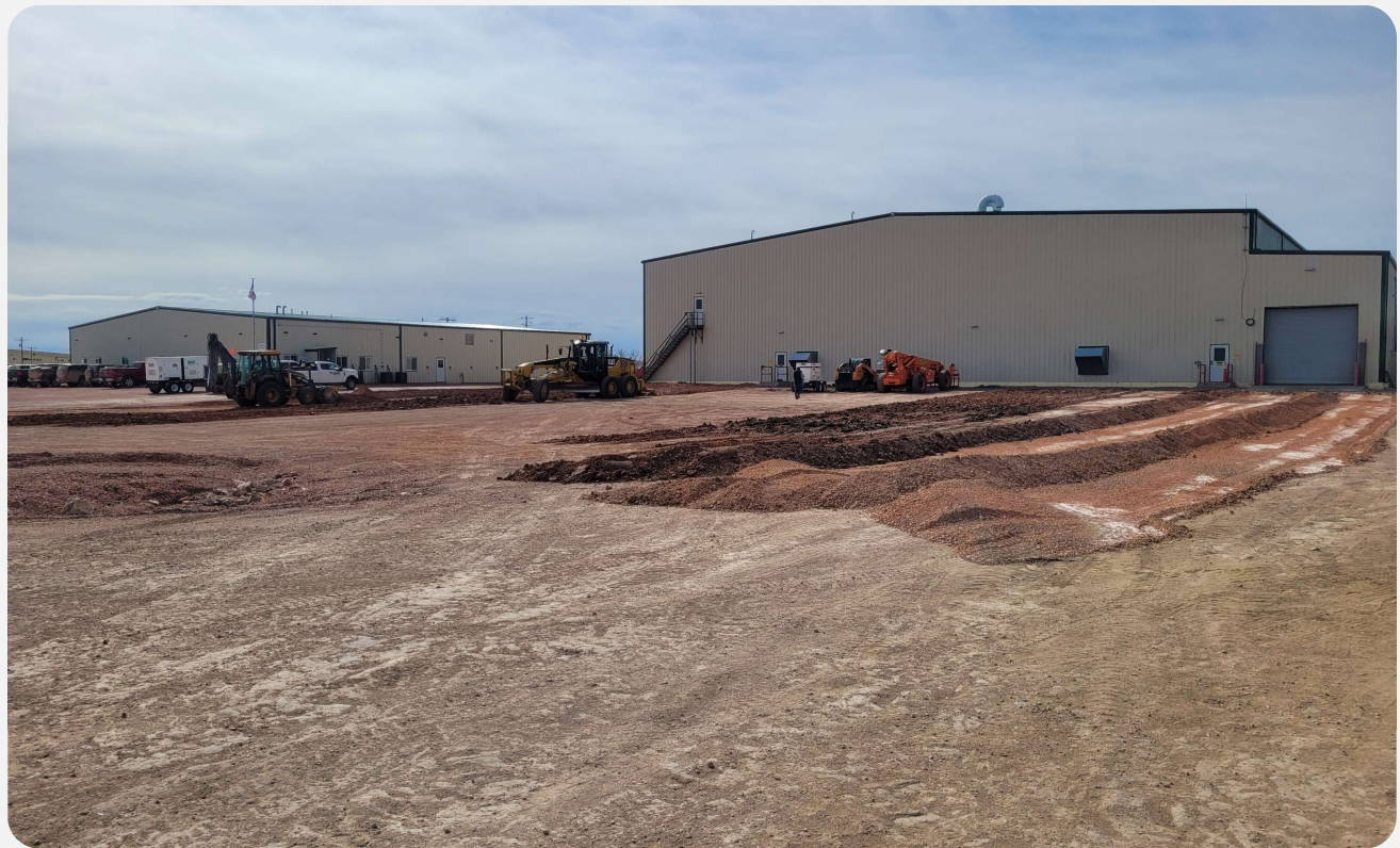
Early Earthworks in advance of Construction
