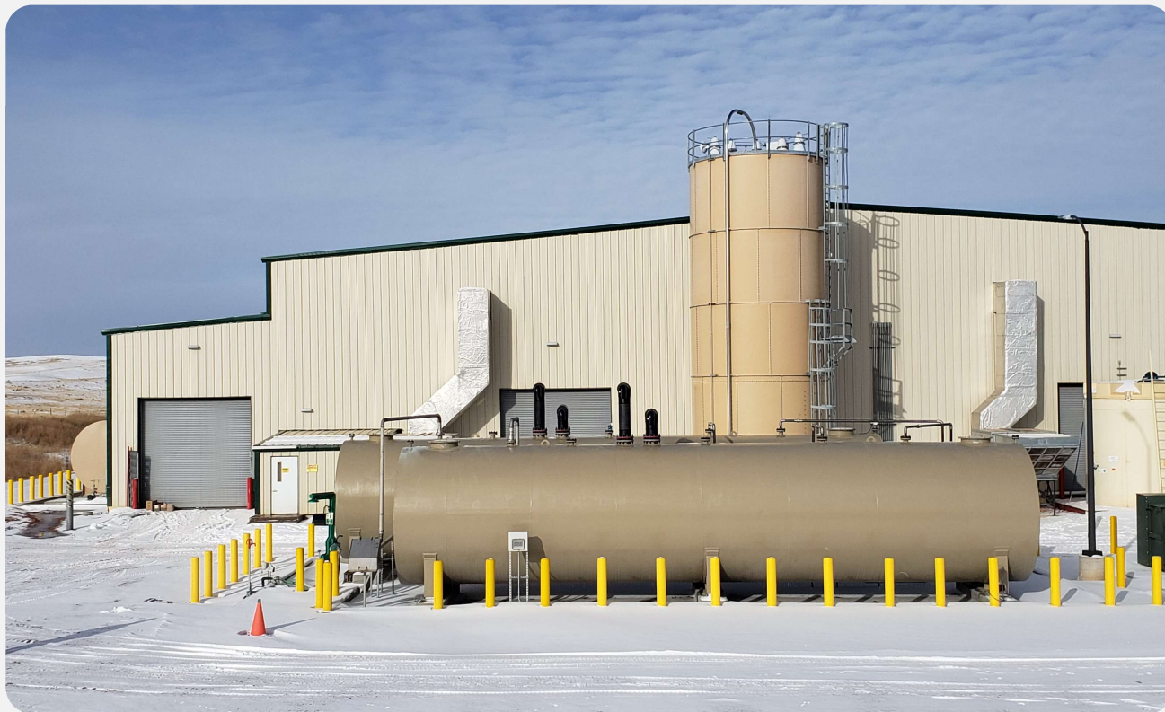
Acid Storage Tank Addition at Lance Satellite Plant
