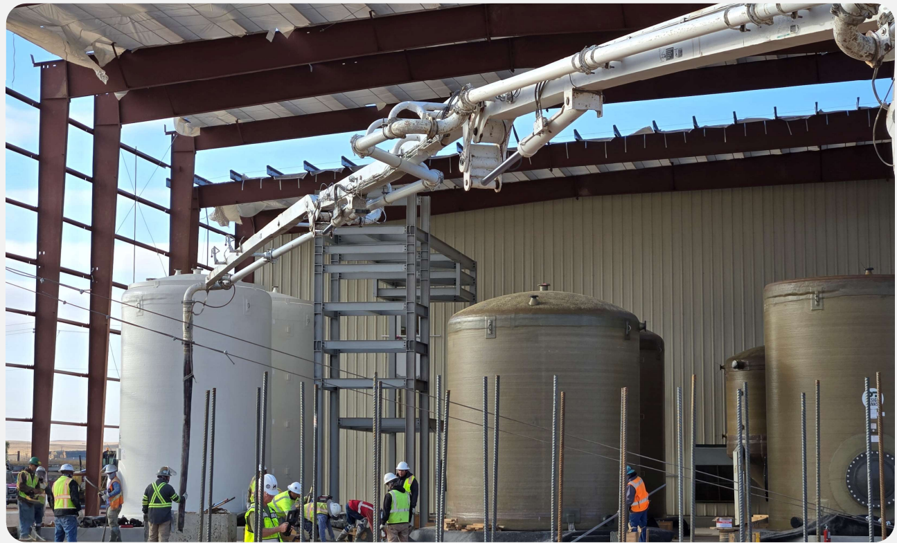
Pouring plant concrete and setting tanks
