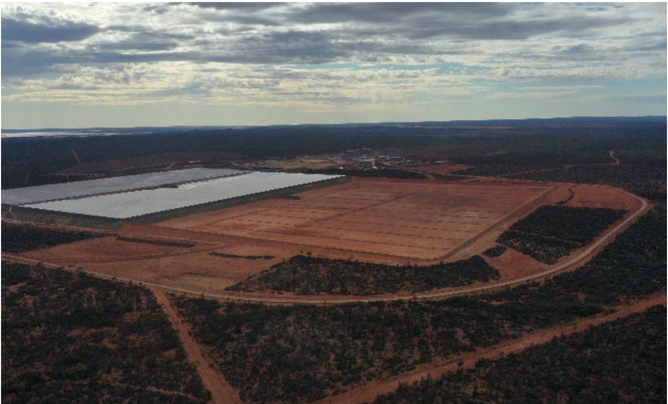
Plate 1 – TSF Cell 4 looking south south-west.
