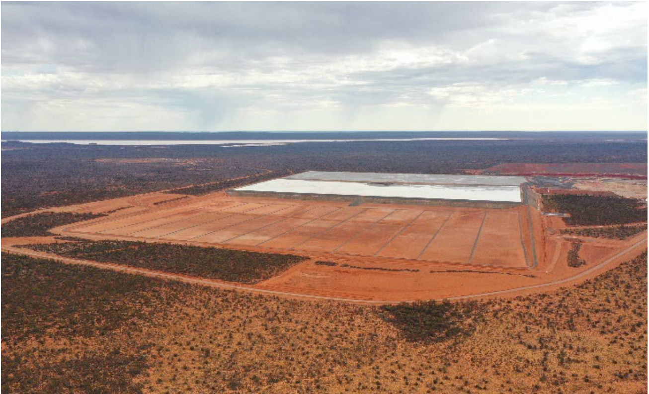
Plate 2 – TSF Cell 4 looking east.
