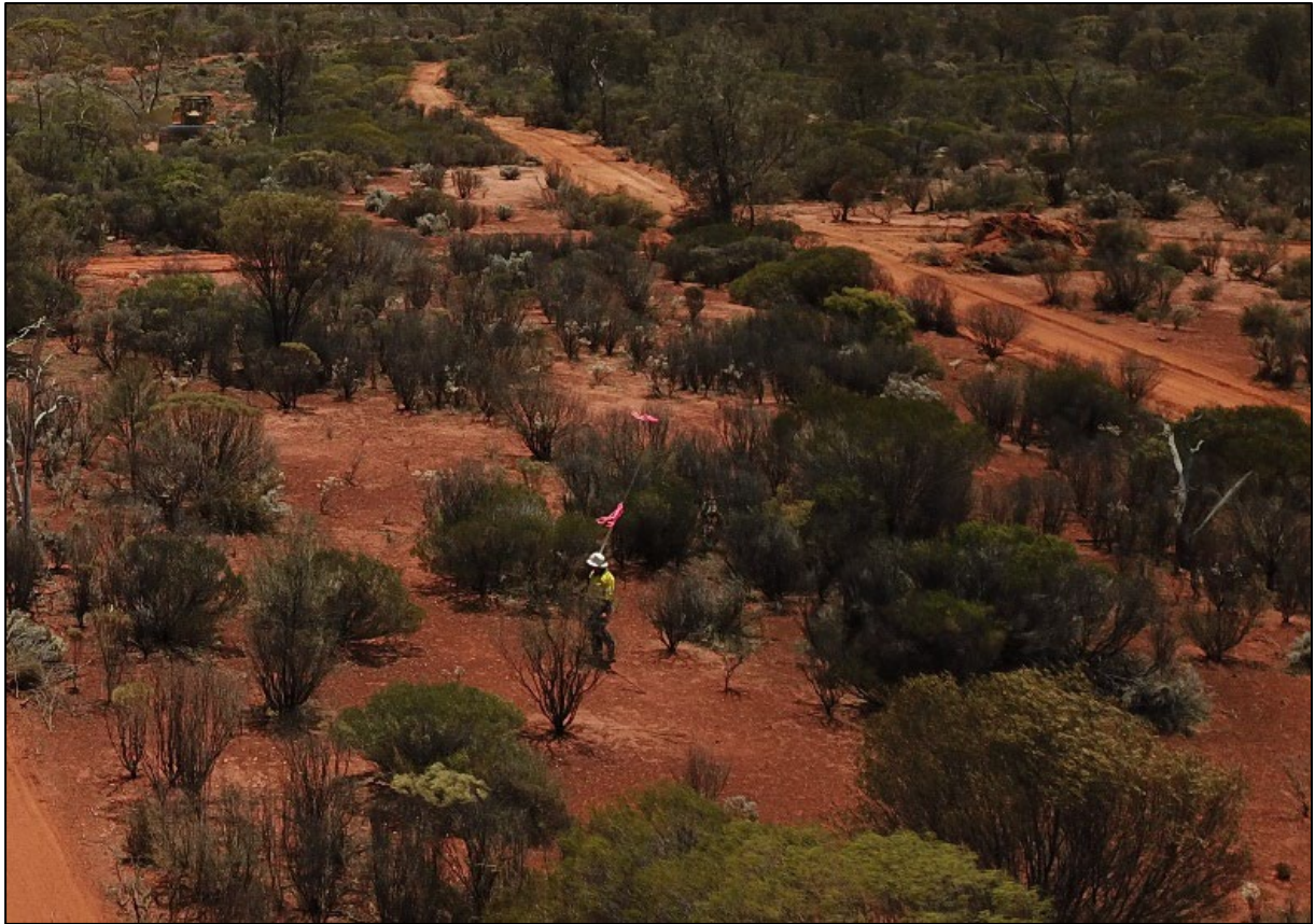
Plate 4 – Fauna spotter walking ahead of dozer during clearing activities.
