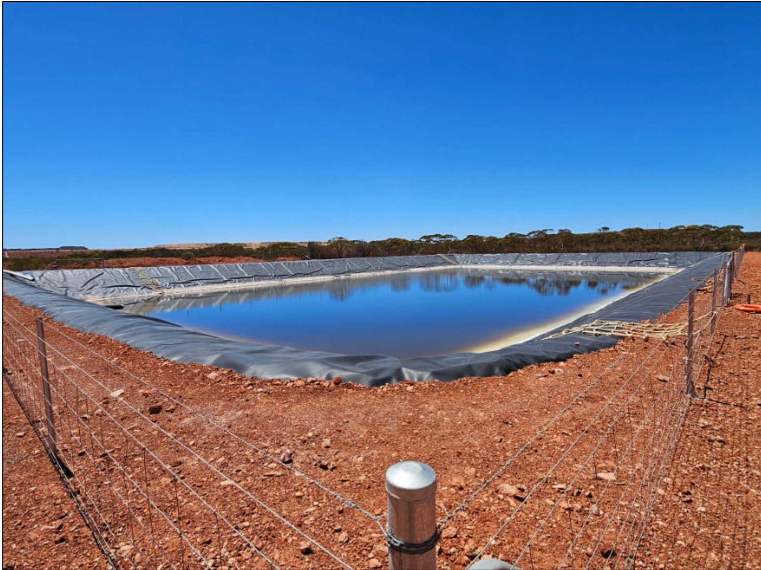
Plate 5 – Fencing and Fauna egress netting around water holding facility
