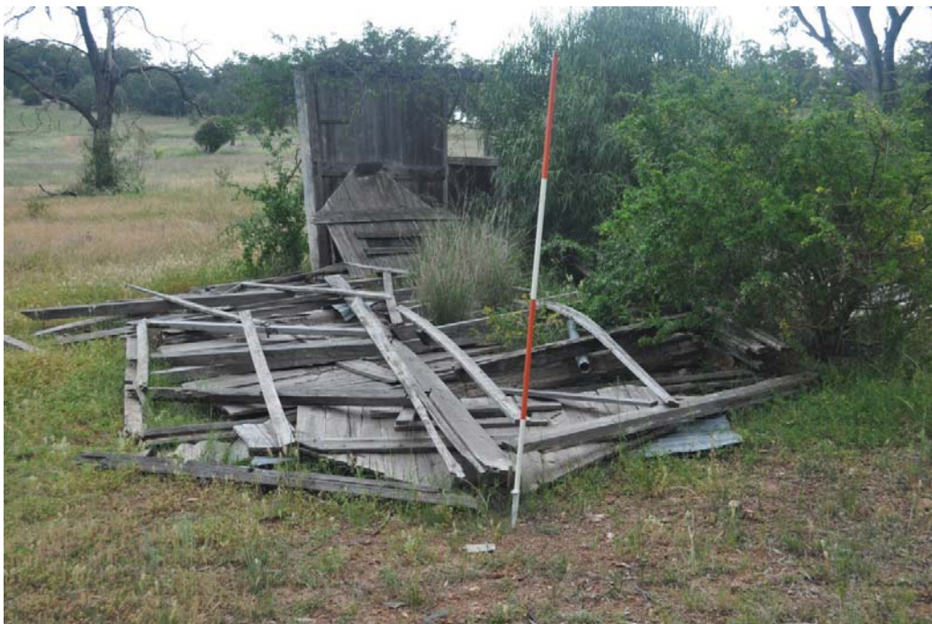
Figure 7: Demolished outbuilding on the site of the Velyama Homestead.
