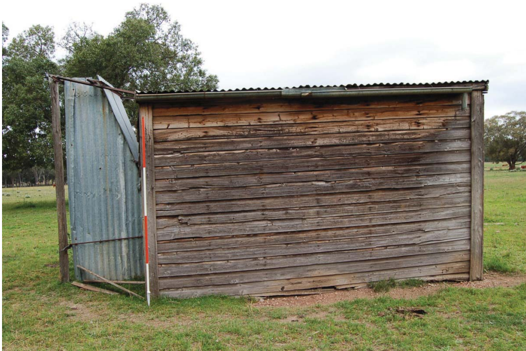
Figure 52: The rear elevation of the Warriahdool 'hut'.
