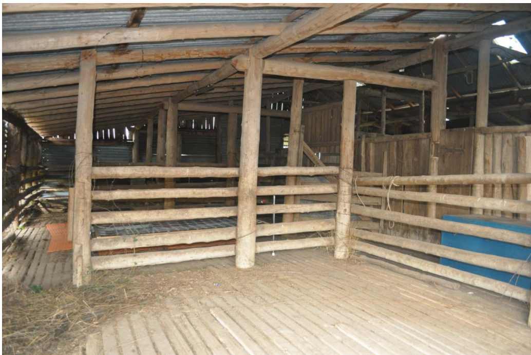
Figure 24: Pens and chutes for sheep constructed of round log timber.
