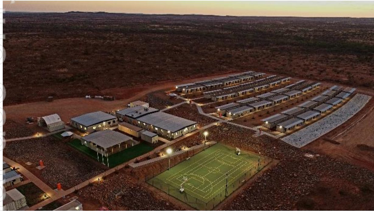
Kurrbili Village - 294 rooms fully commissioned with medical centre, sports court, shop, dry and wet mess.
