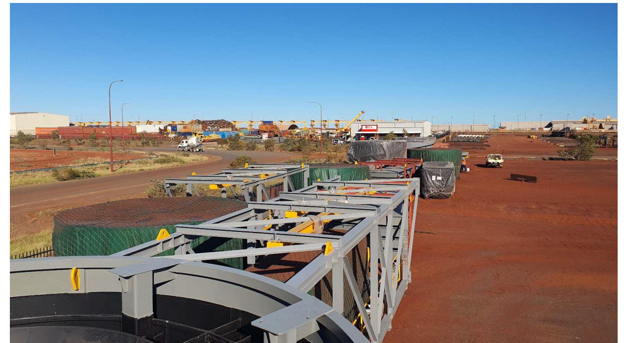
Flotation Cells & Structural Steel ready for installation.
