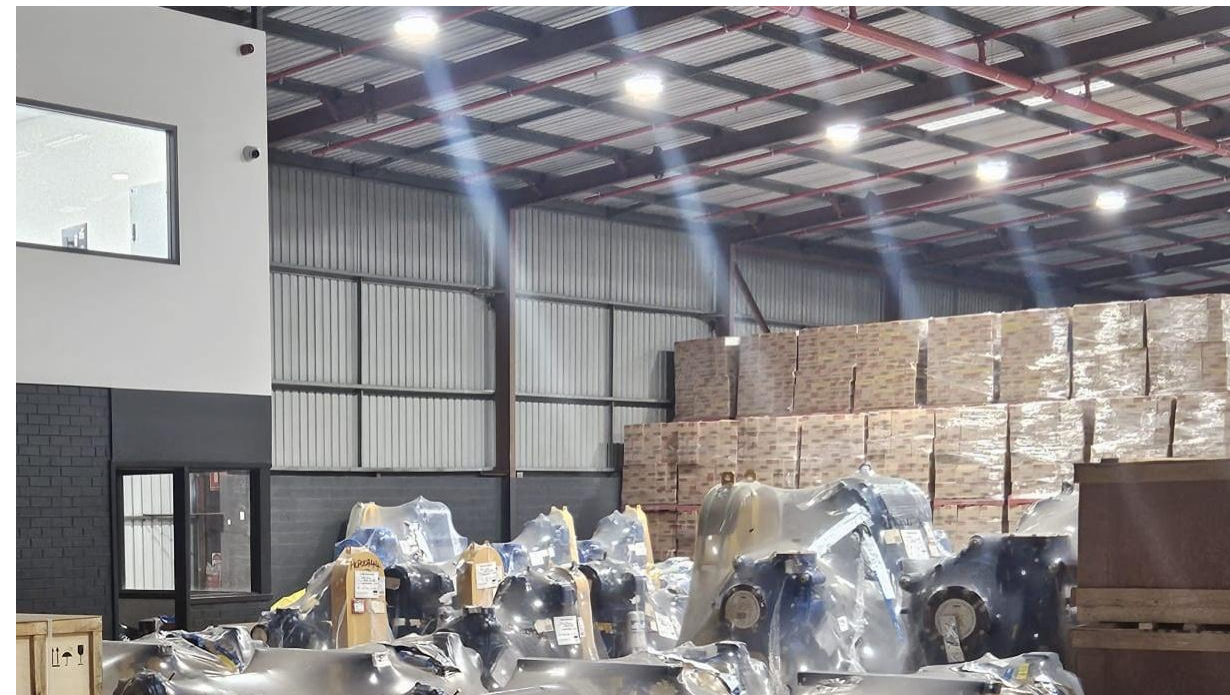
Equipment - Long Lead Equipment in WA and in storage ready for installation.
