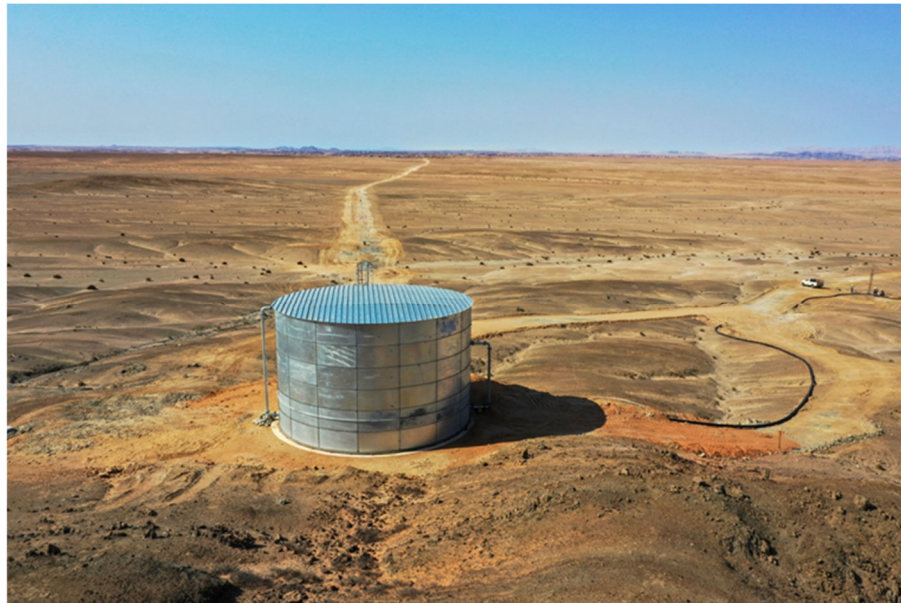
Figure 2 – The water reservoir completed in July 2024 has a diameter of 11.7m and can hold up to 700m 3 of water
