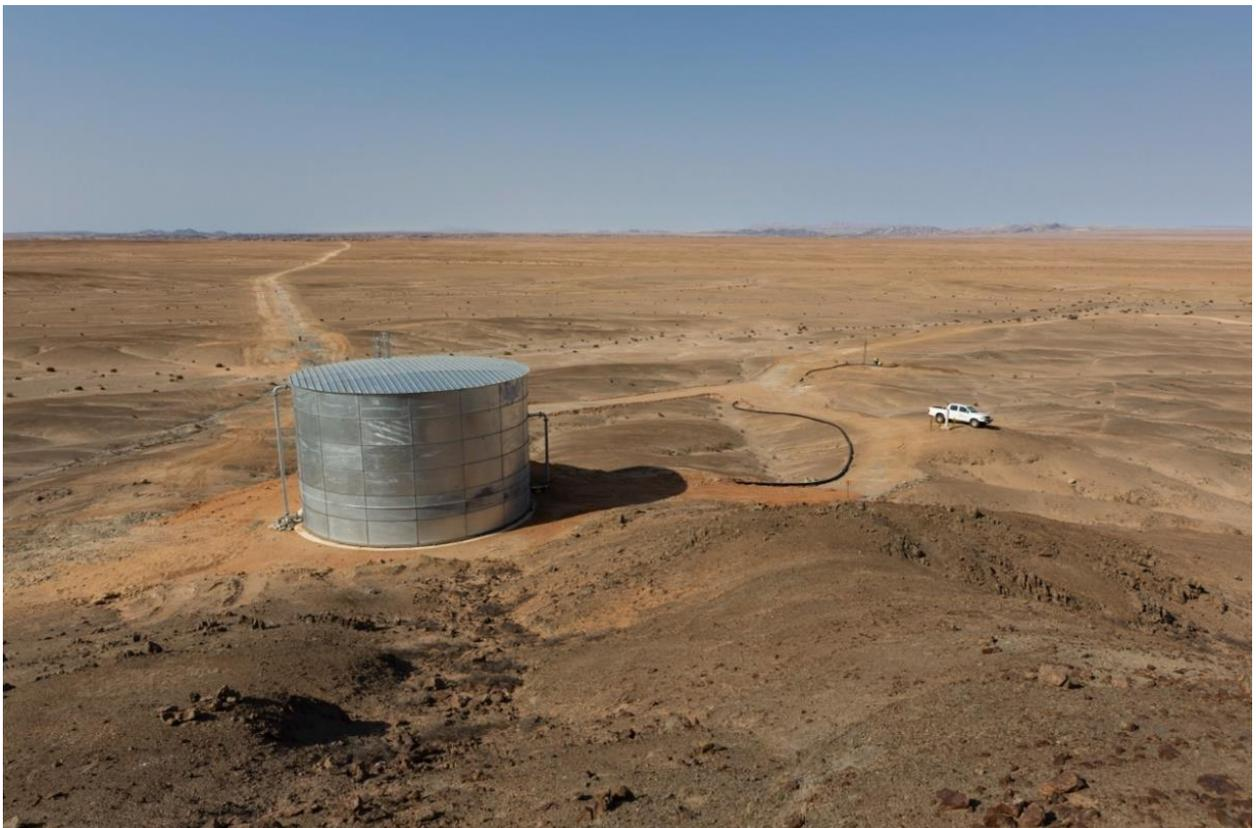
*Figure 3: Completed construction water reservoir delivering 700m<sup>3</sup> storage volume*
