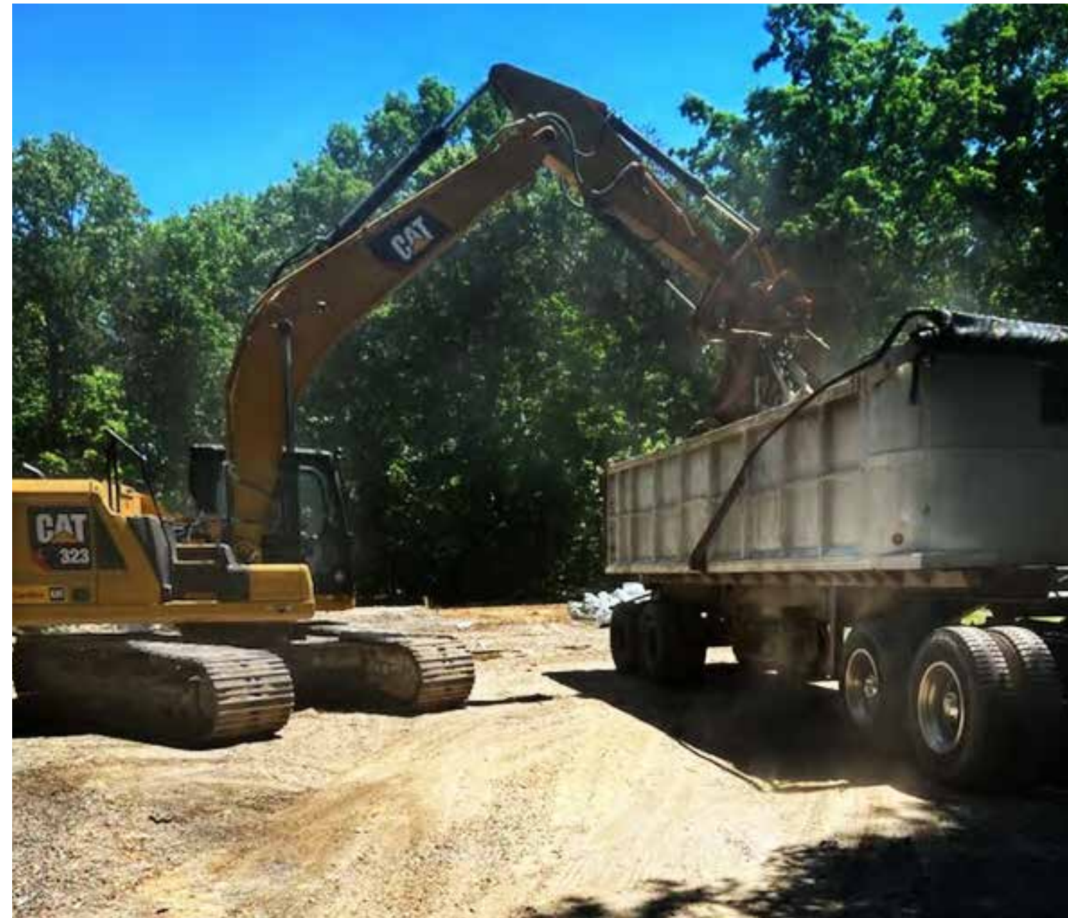
↑ Since beginning geological activities at Carolina Lithium, we have worked closely with S.C. Lovelace and Sons, a local contractor experienced in the mining industry. Lovelace performs a range of earthworks, including reclamation activities when homes are purchased and no longer needed on the project site.
