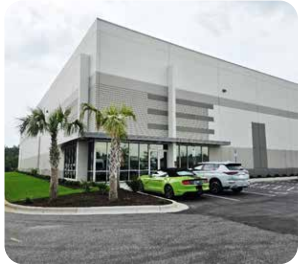
GLE HQ Facility – Wilmington, NC
