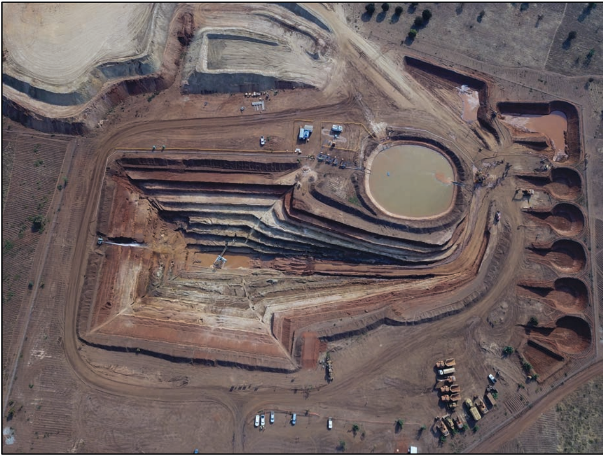
Figure 7: Overview of the hydraulic mining trial
