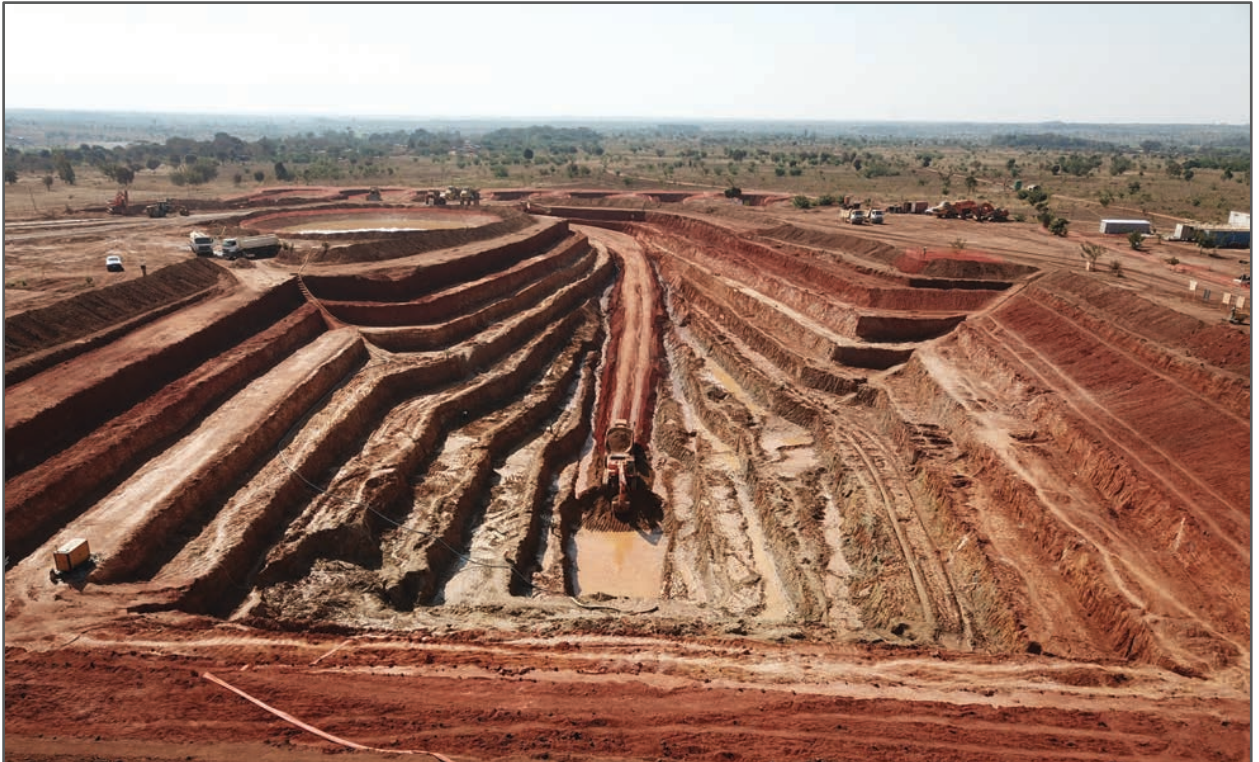
Figure 5: Kasiya Pilot Phase Test Pit mined to 20 metres depth
