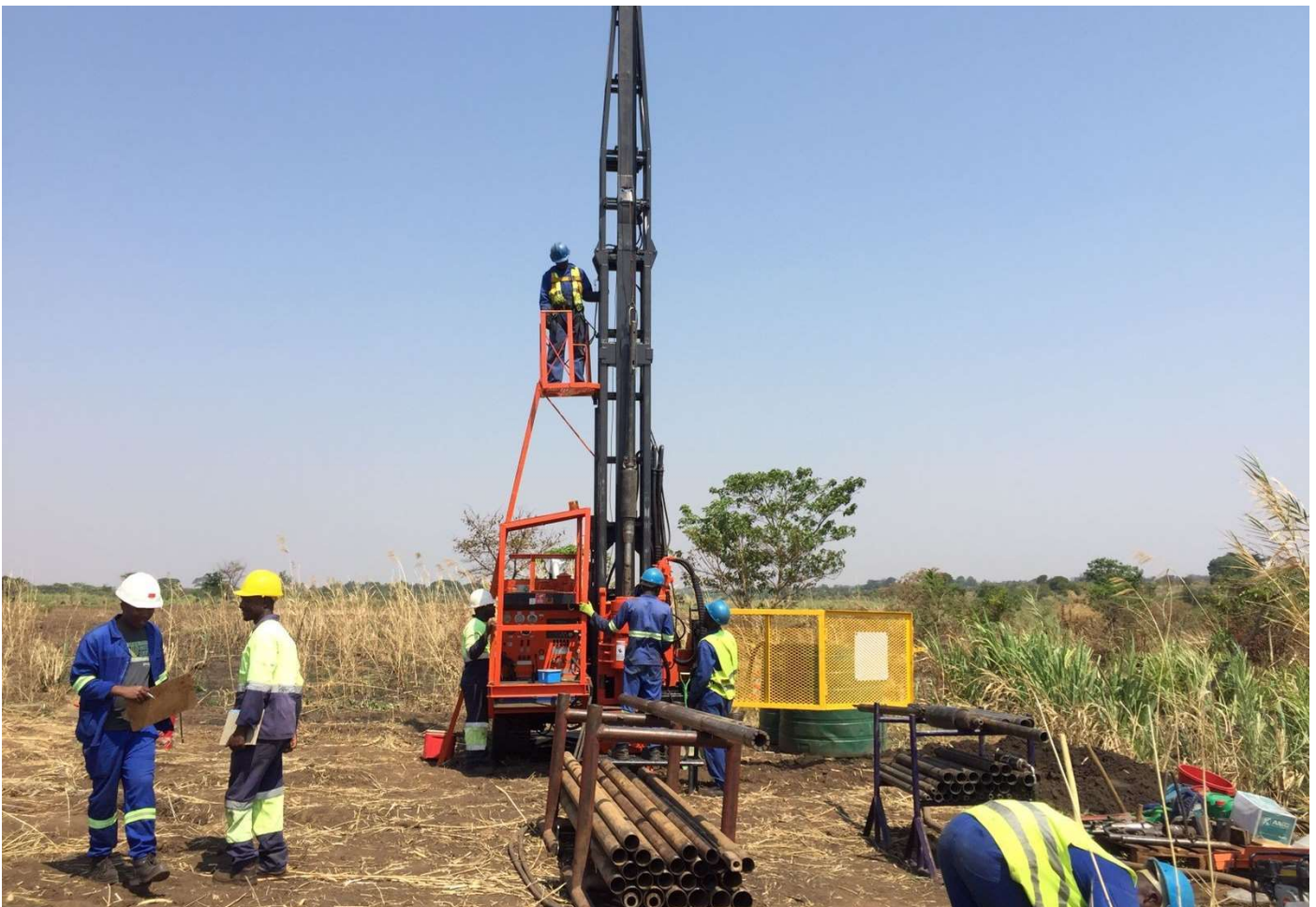
Figure 11: Water drilling underway at Kasiya
