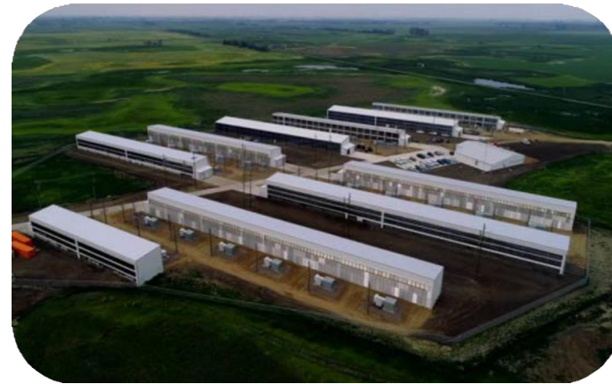
Ellendale, North Dakota Facility 180MWs
