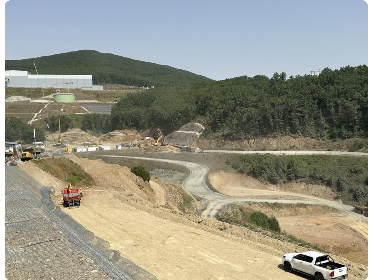
Water treatment plant location
