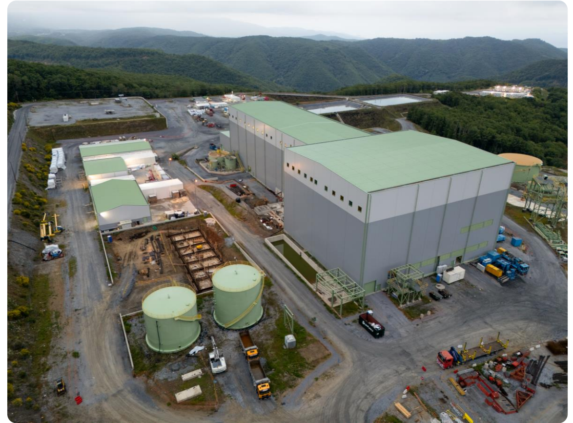
May 2024: aerial view of mill building.
