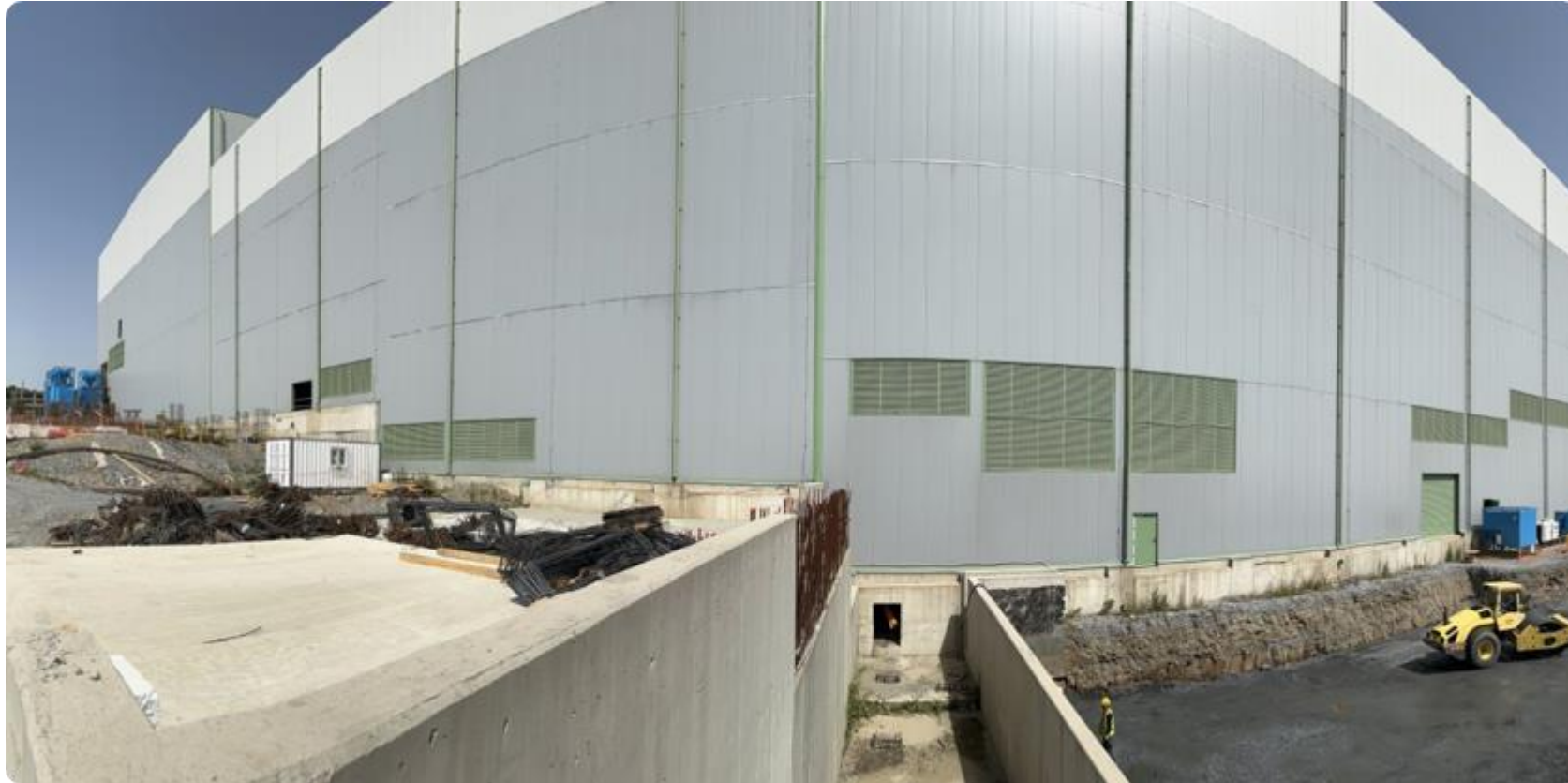
East side of main process plant building
