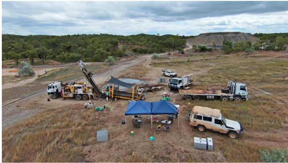
Figure 13. Drilling hold D15 in May 2024
