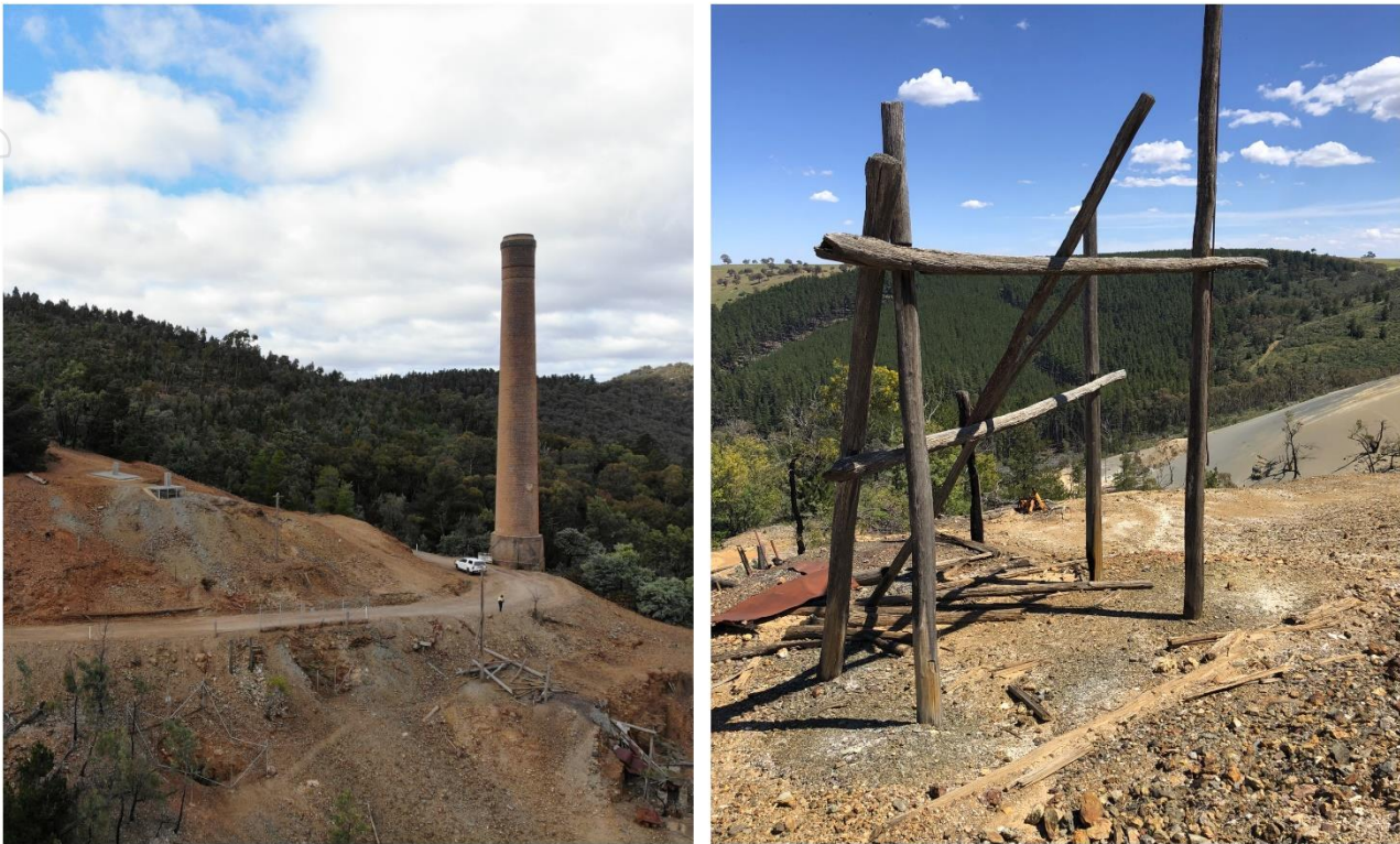
Figure 7: Old workings at the Lloyds Copper Mine at Paterson Resources Burruga Copper-Gold Project in NSW
