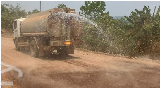
Figure 29 | Dust suppression on community road
