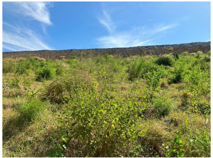
Figure 18 | Okvau waste rock dump under rehabilitation
