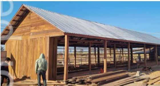
Figure 26 | New roof on school building
