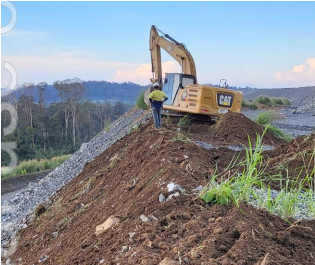
Figure 19 | Okvau batter/berm trial
