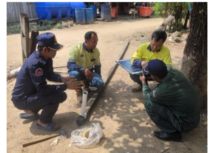
Figure 28 | Installing roadside lighting
