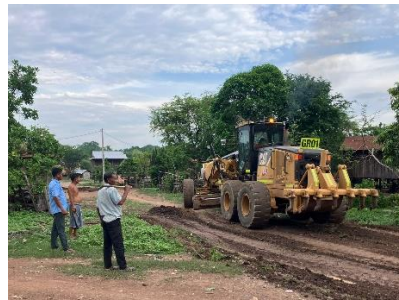
Figure 27 | Village road upgrades
