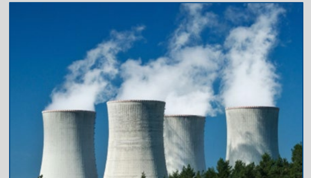
Nuclear spares for public utility company
