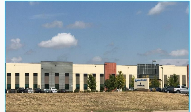
Applied Control Equipment – Denver, CO
