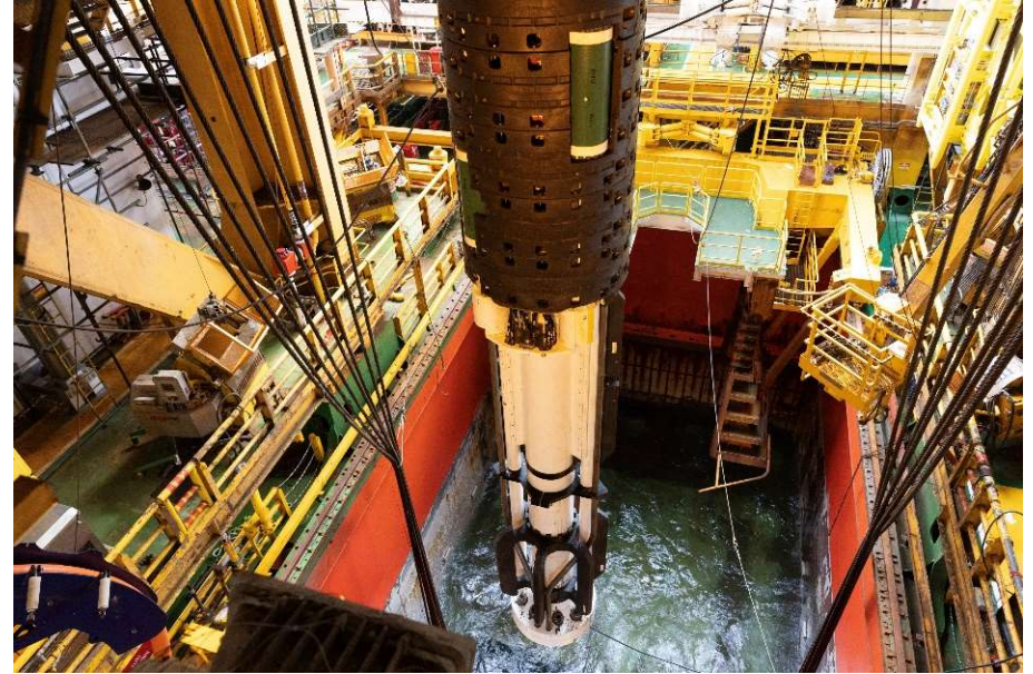
Shown above: Oil States Managed Pressure Drilling (MPD) Integrated Riser Joint Aboard the West Polaris Deepwater Rig
