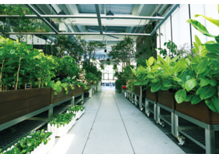
Greenhouse that uses waste heat
