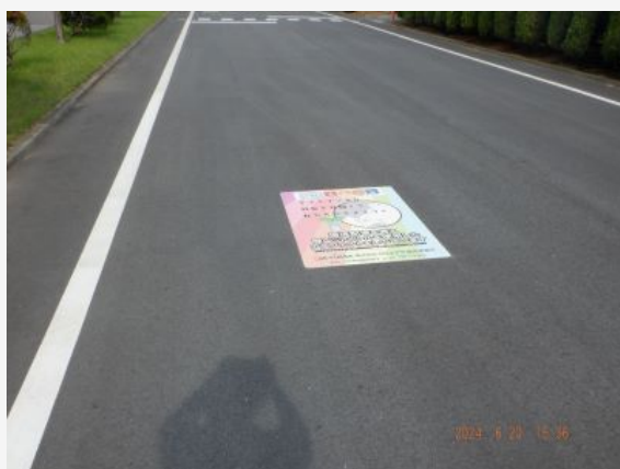
Environmentally considered road pavement on the premises (Gunma Plant)
