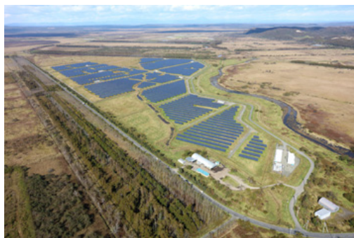
Overall view of Kushiro Toritouchi Wildland Photovoltaic Generation Plant
