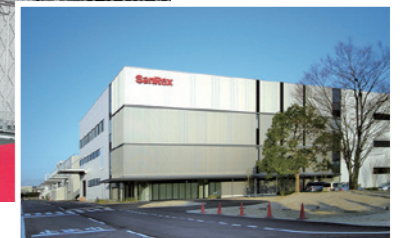
New building completed at the Shiga Plant
