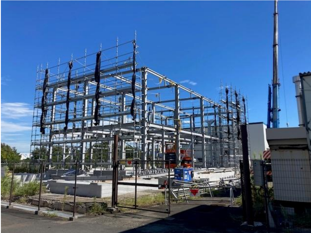
Figure 3: Demonstration Facility Construction
