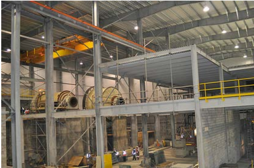
Rubicon Minerals photo of Phoenix mill construction, September 2014
