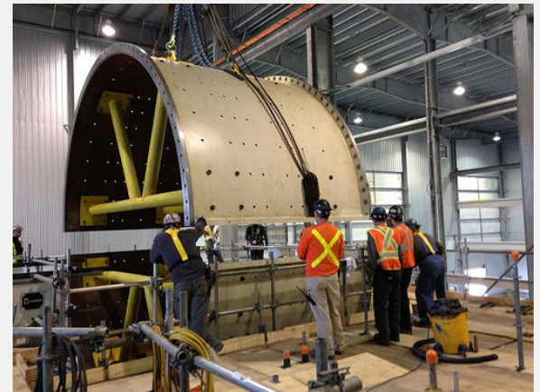
Phoenix mill construction, August 2014
