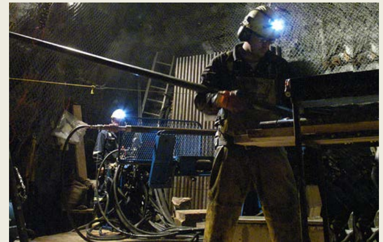
Underground development at Phoenix, 2014
