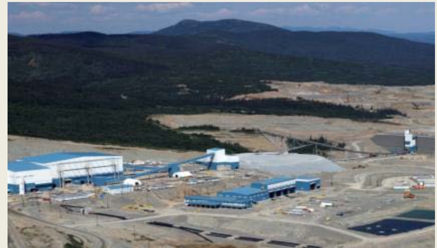
Mt. Milligan Facilities, July 2013
