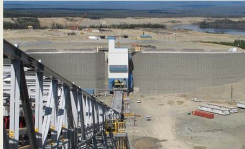
Mt. Milligan Primary Crusher
